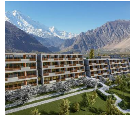
Hunza Serena Hotel (Under Construction)
