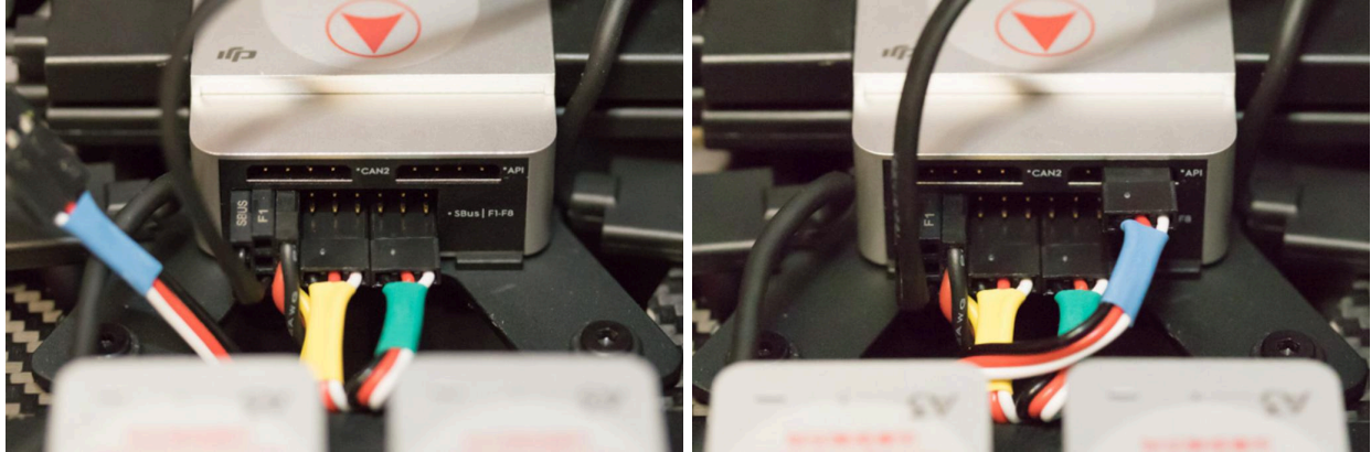
Figure 9.2d: Three connectors installed.
