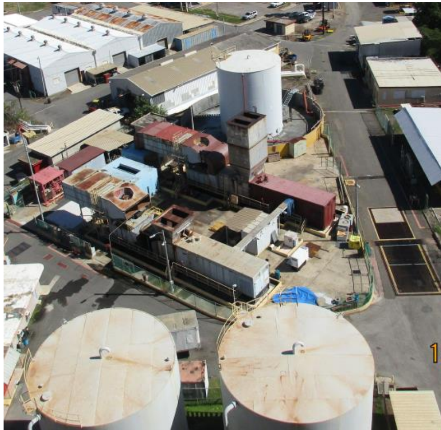
Figure 3-1 — Black Start Gas Turbines
