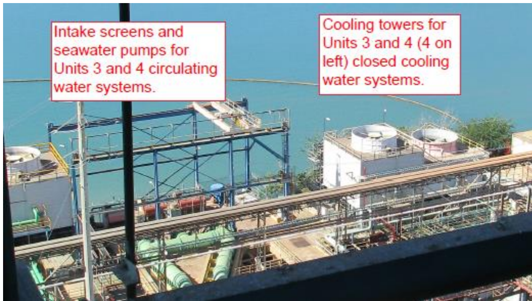
Figure 2-2 — Units 3 and 4 Seawater Intake and Closed Cooling Tower
