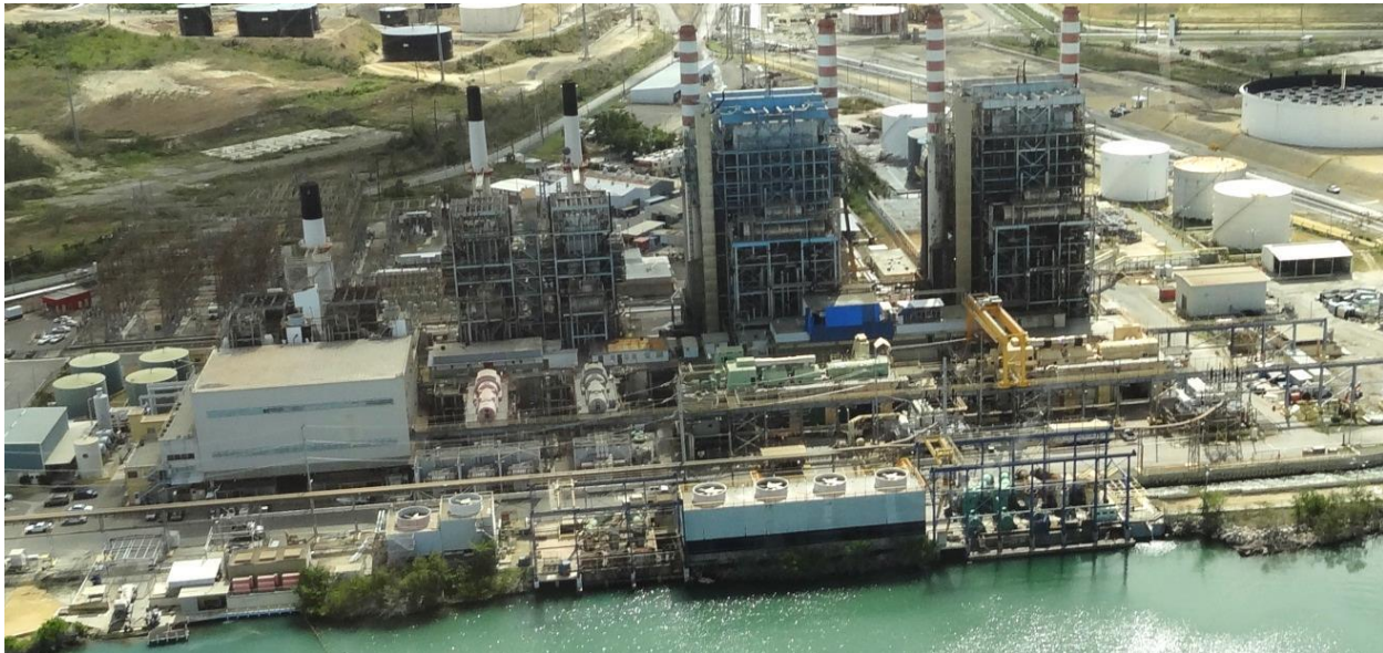
Figure 1-3 — Costa Sur Steam Plant
