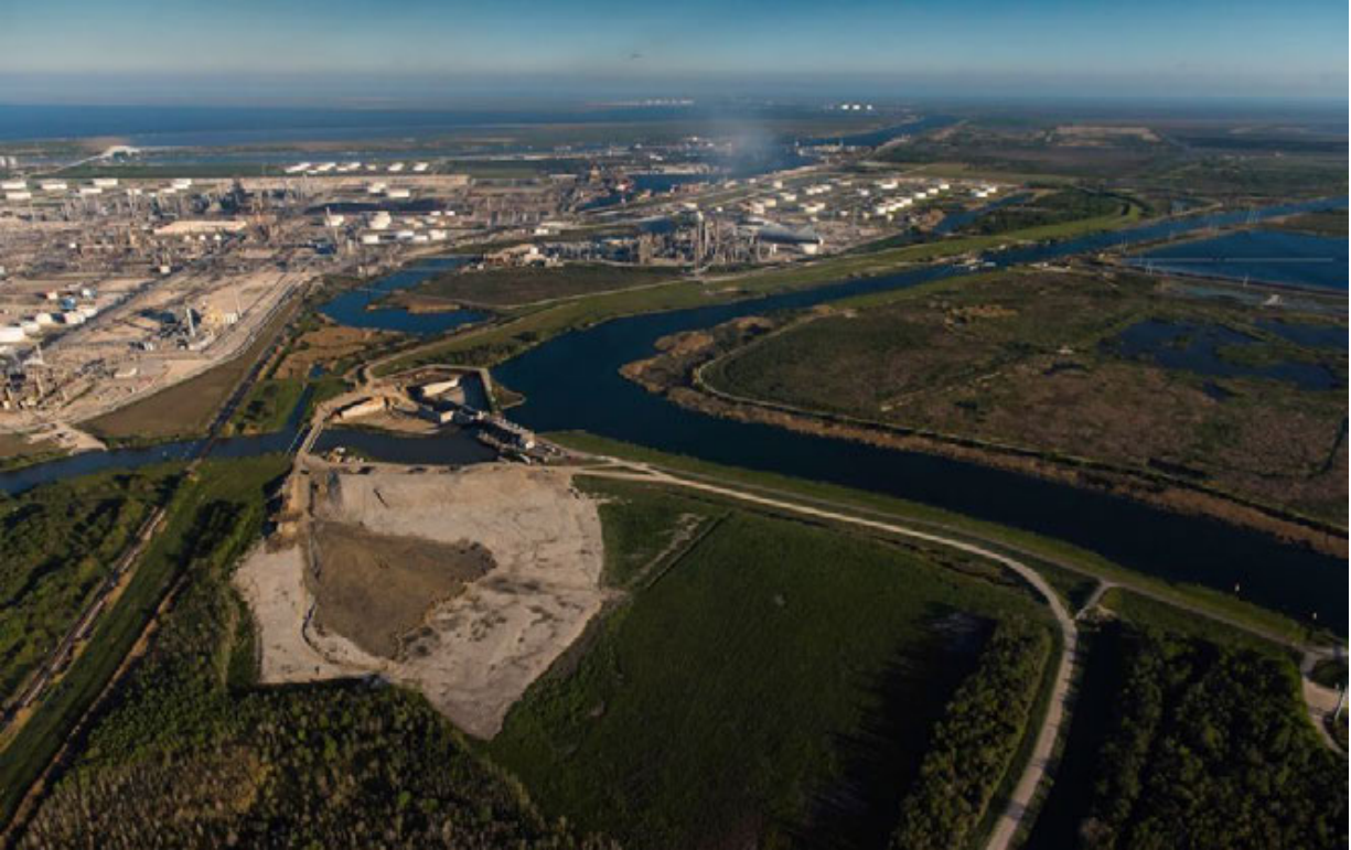
Chevron Phillips petrochemical plant near the Valero Refinery. Copyright Garth Lenz.
