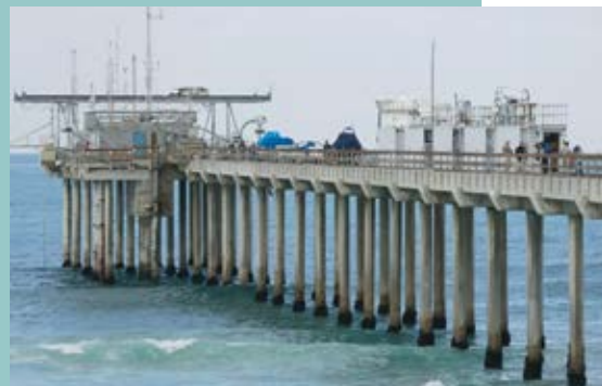
Equipment lines the Ellen Browning Scripps Memorial Pier for the Eastern Pacific Cloud Aerosol Precipitation Experiment project. Credit: K.C. Alfred / The San Diego Union-Tribune
