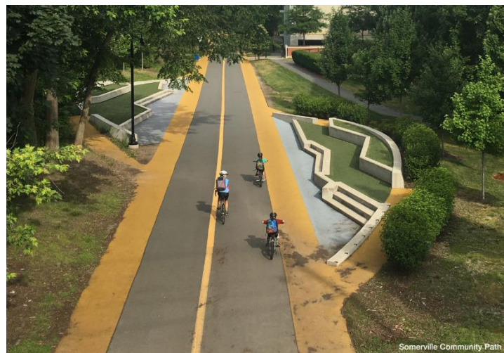
Figure 10: Speed Segregated Multi-use Path
