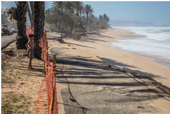
Image: Erosion of bike path along Sunset Beach on O'ahu (Credit: Rafael Bergstrom).
