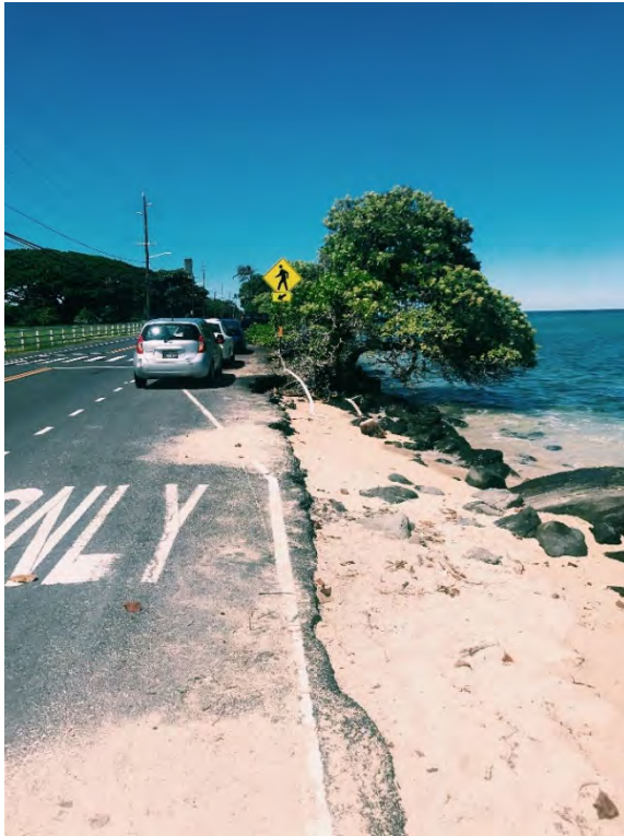
Image: Shoreline encroaching on a roadway on O'ahu (Credit: Abbey Seitz)
