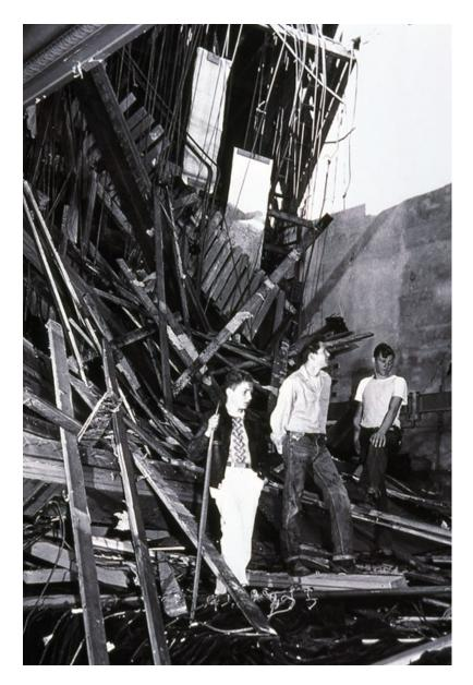
**Figure 3.** Photograph from the Seattle Times showing damage to Puyallup High School during the 1949 Olympia earthquake.
