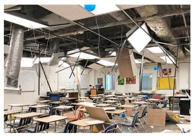
**Figure 10.** Nonstructural earthquake damage to a high school in Anchorage, Alaska, from the 2018 M7.0 Anchorage Earthquake (Photo by Reid Middleton, Inc.).
