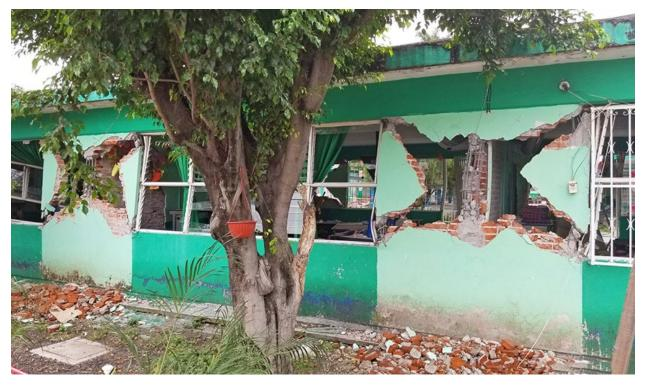
**Figure 9.** Structural earthquake damage to a primary school in central Mexico from the 2017 M7.1 Central Mexico Earthquake (Photo by Reid Middleton, Inc.).
