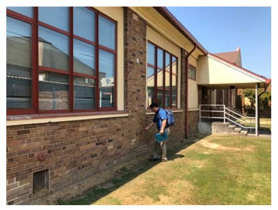
Figure 8. Structural Engineer inspects a school building using the ASCE 41-17 Tier 1 checklist.
