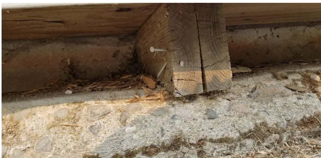
Figure 1-9. Example of foundations and minor deterioration of concrete
