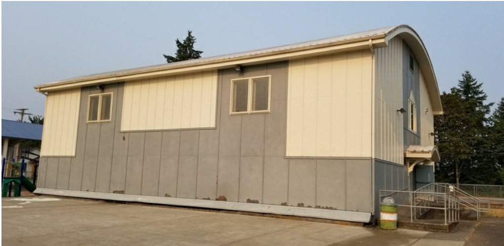
Figure 1-1. East facade of building
