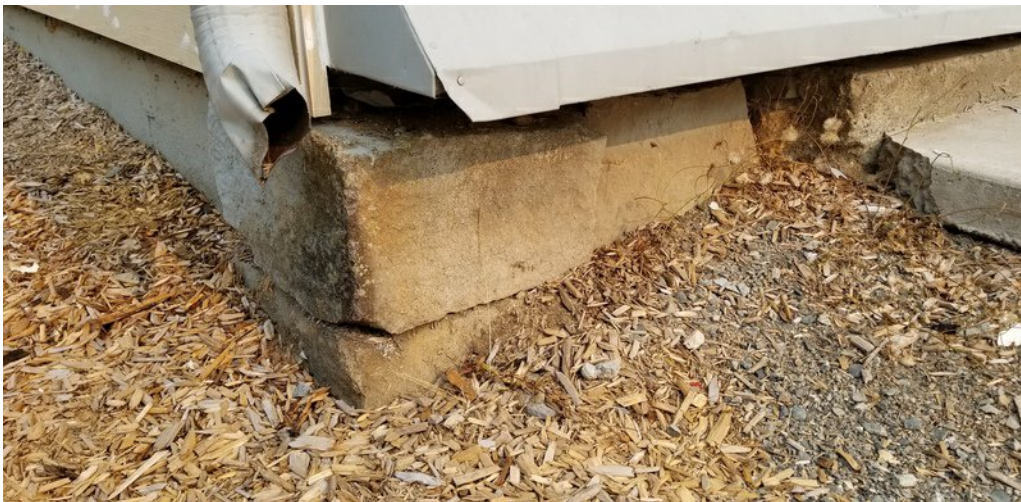
Figure 1-2. Example of foundation condition (SE corner of building)
