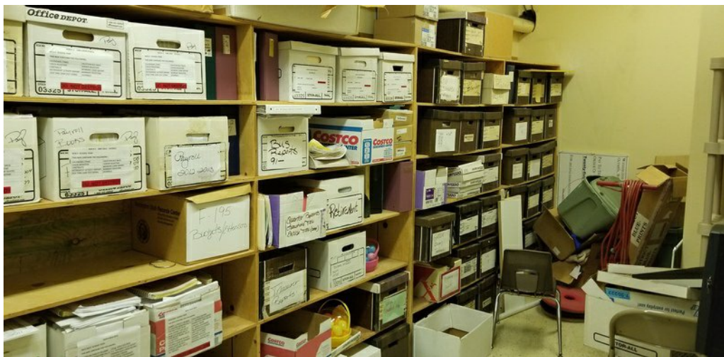
Figure 1-7. Fall prone content and shelving that is not adequately braced
