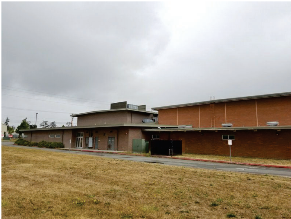
Figure 1-2. Auxiliary and existing gym
