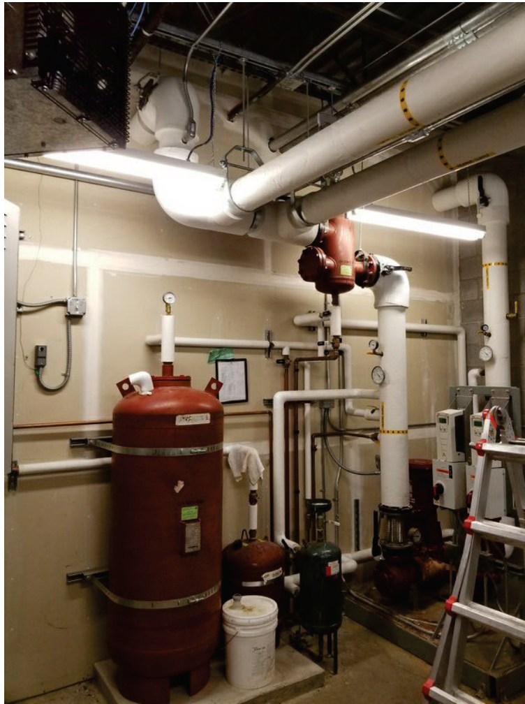
Figure 1-5. Braced mechanical system
