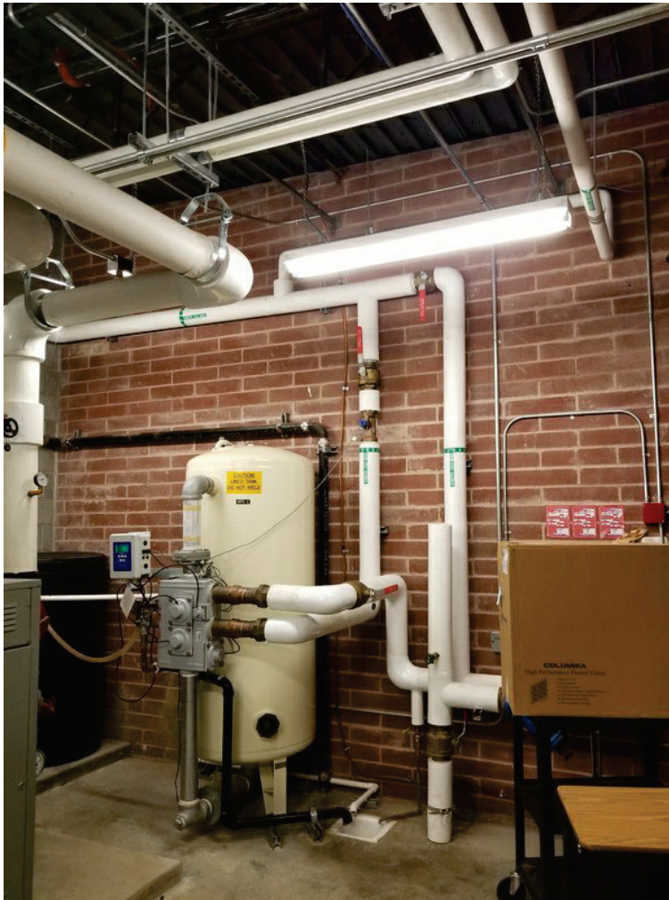
Figure 1-6. Braced mechanical system
