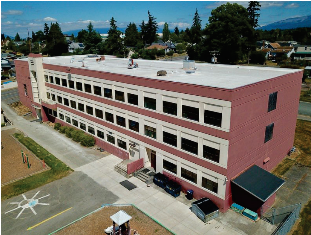
Figure 1-8. Exterior west side of building.
