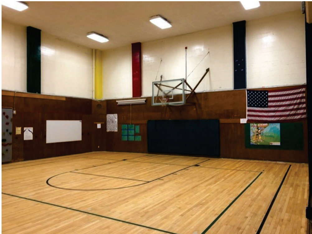
Figure 1-4. Basement level gymnasium with cast-in-place concrete walls and pilasters. The performing arts space is on level 3 above the gym.
