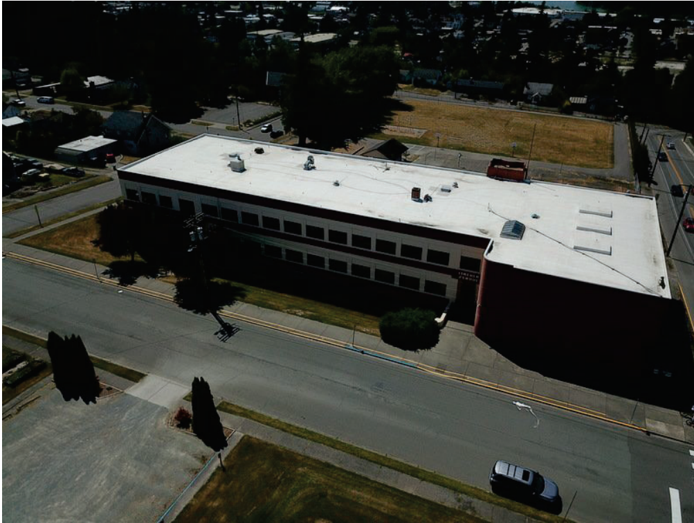
Figure 1-10. Exterior east side of building.
