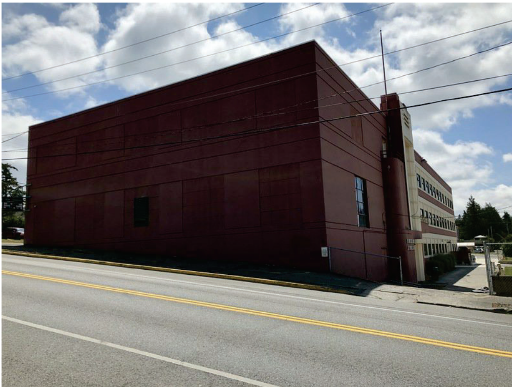
Figure 1-7. Exterior north side of building. Note high bay gymnasium with a performing arts space above the gym.
