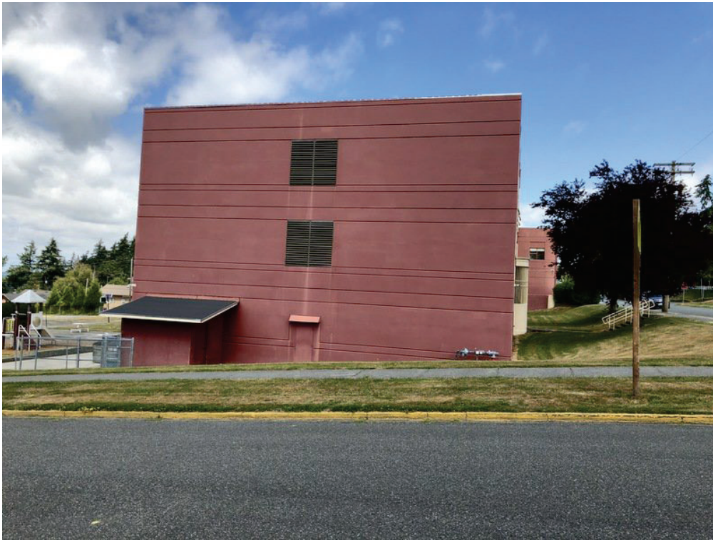
Figure 1-6. Exterior south side of building. Note concrete exterior walls and gently sloping site.
