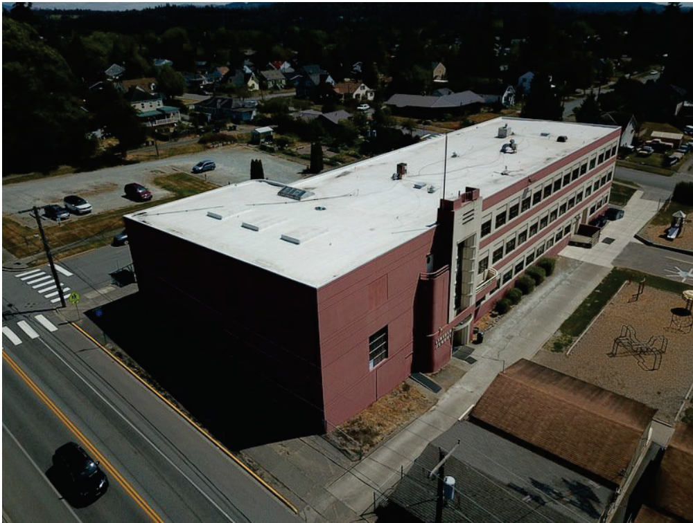
Figure 1-9. Exterior northwest corner of building.
