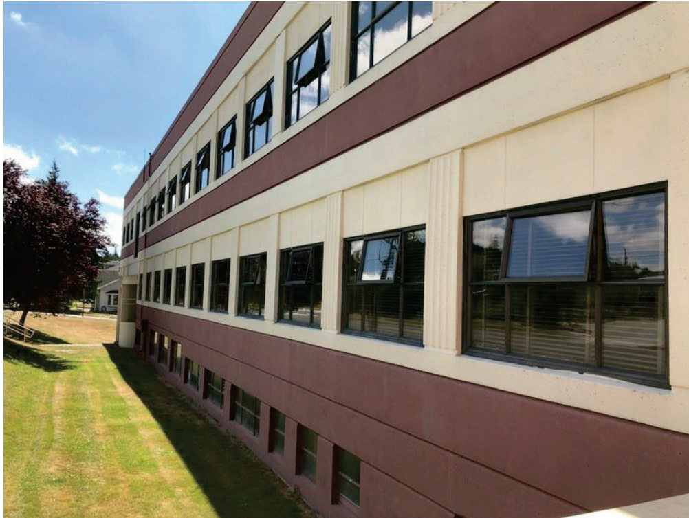
Figure 1-1. East elevation concrete wall. Notice short wall piers at lowest level.
