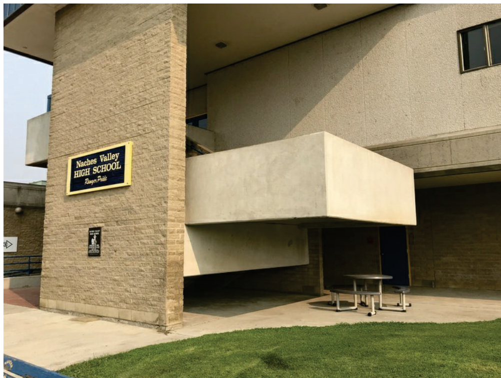
Figure 1-2. Naches Valley HS Classroom Bldg exterior entry stair
