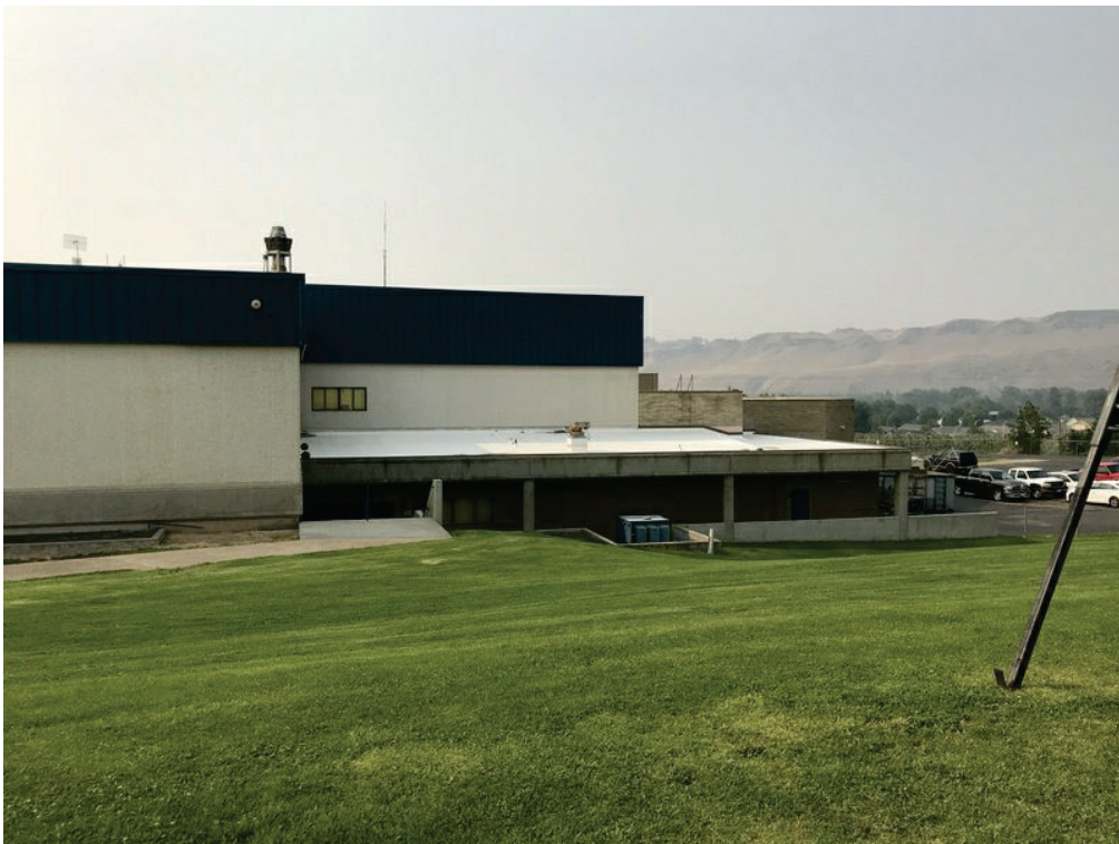
Figure 1-4. Naches Valley HS Classroom Bldg North wall
