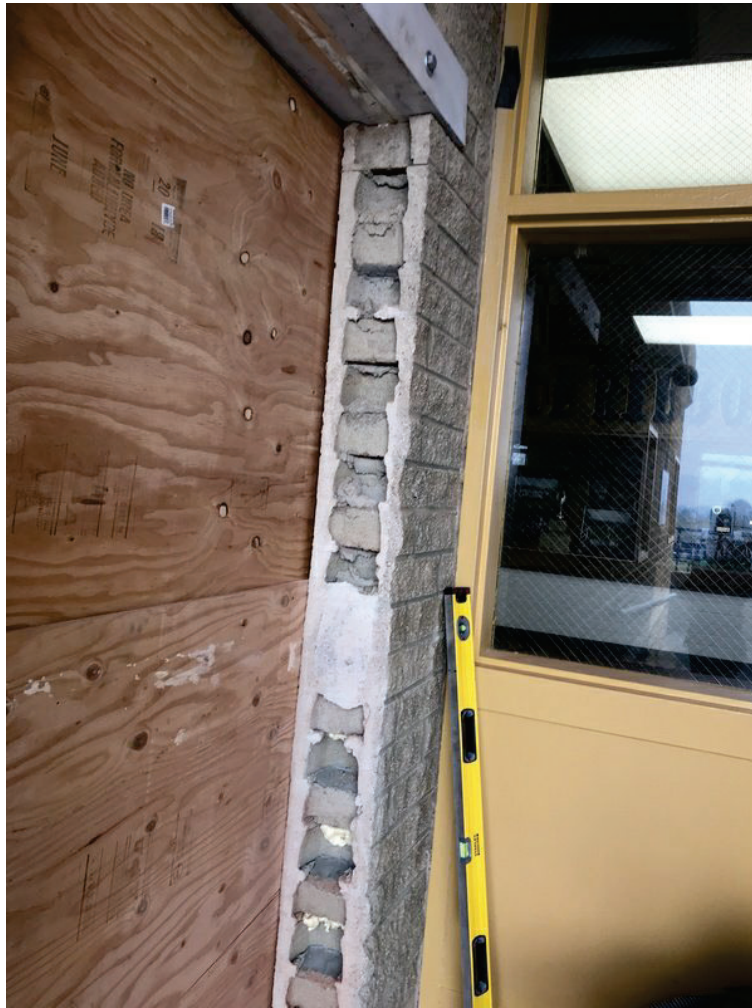
Figure 1-7. Naches Valley HS Classroom Bldg - new door opening exposes wall construction
