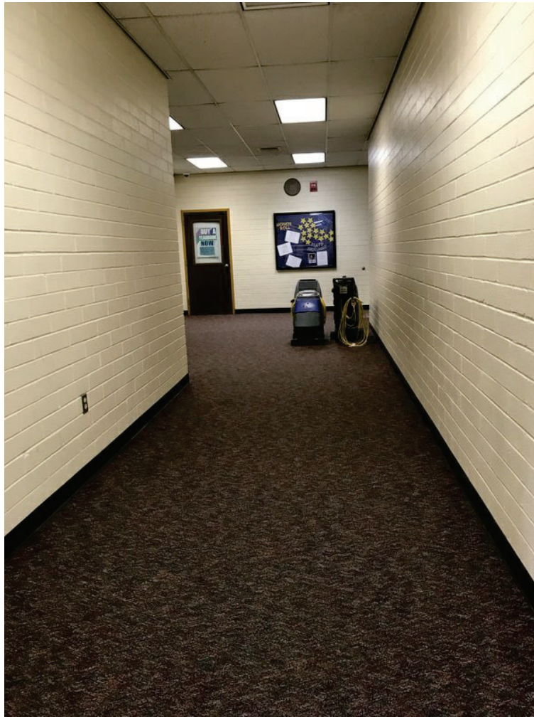
Figure 1-8. Naches Valley HS Classroom Bldg hallway (cmu construction)
