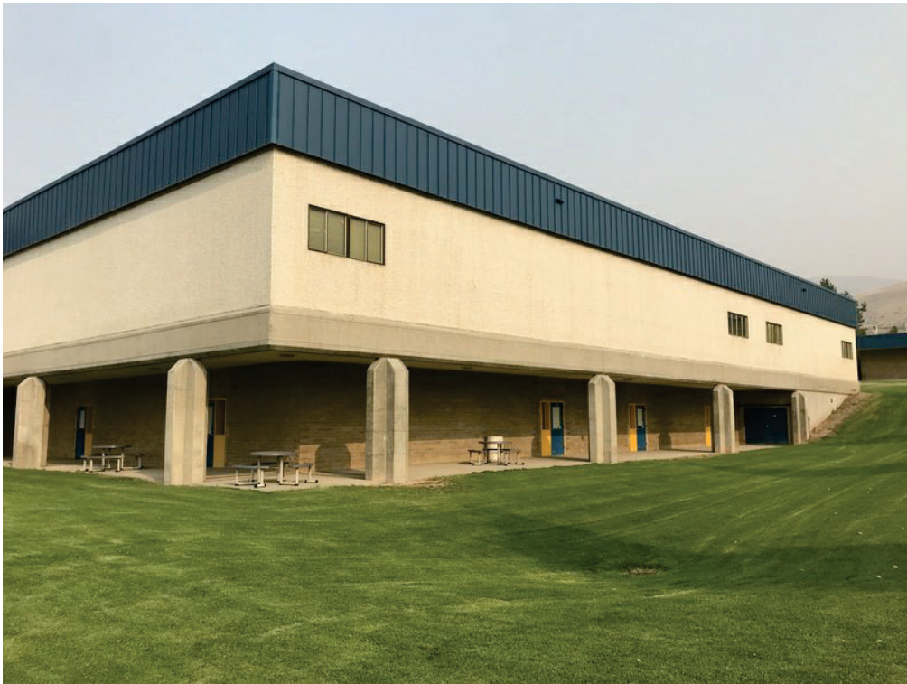
Figure 1-3. Naches Valley HS Classroom Bldg SE corner
