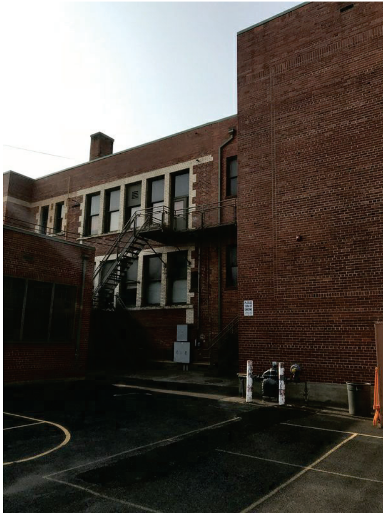
Figure 1-8. View from northwest corner of building, URM chimney can be seen
