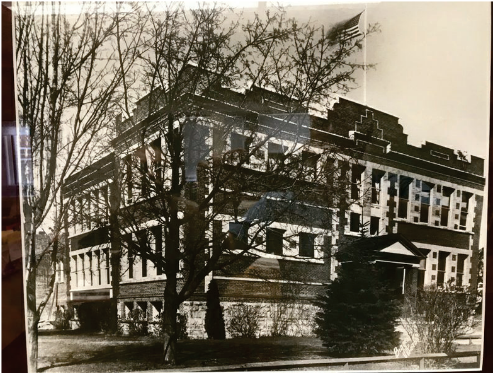
Figure 1-10. Original photo from SE corner of building showing original taller parapet configuration.
