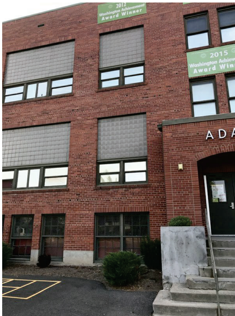
Figure 1-9. West elevation/entry showing infill glass block above windows
