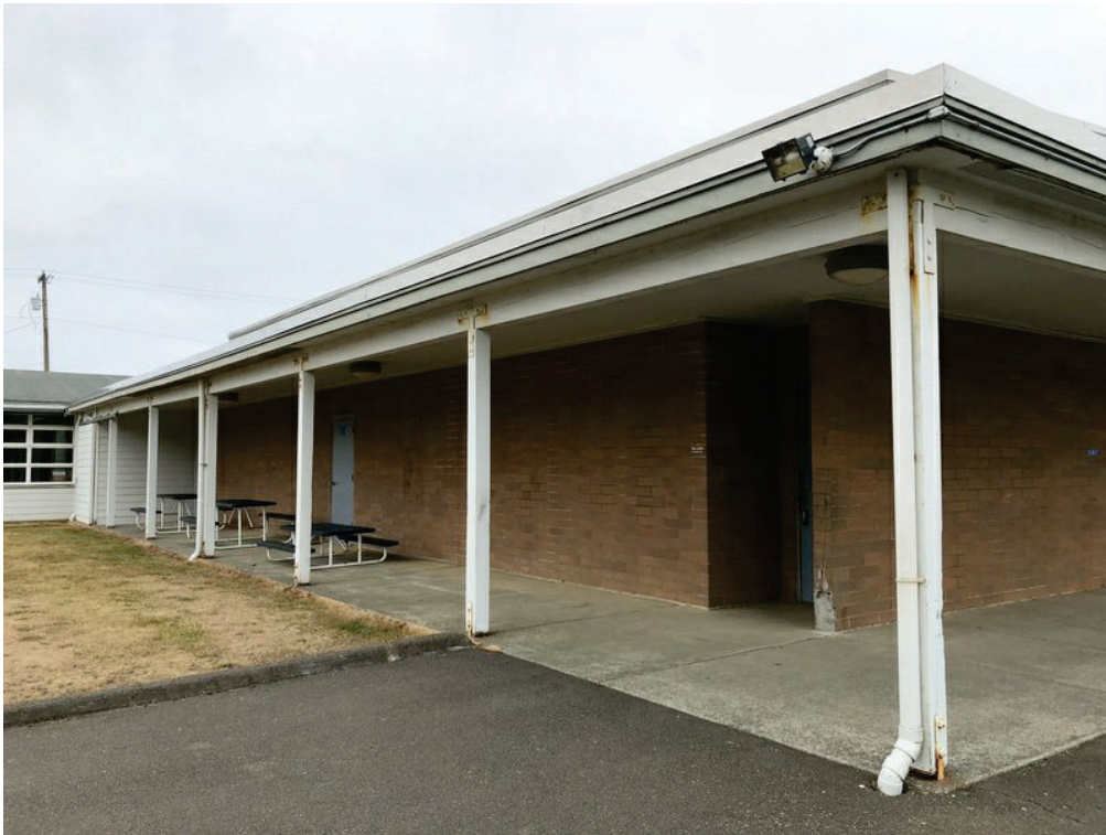
Figure 1-5. South masonry wall and canopy
