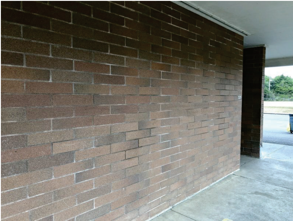
Figure 1-7. Brick masonry wall at south elevation
