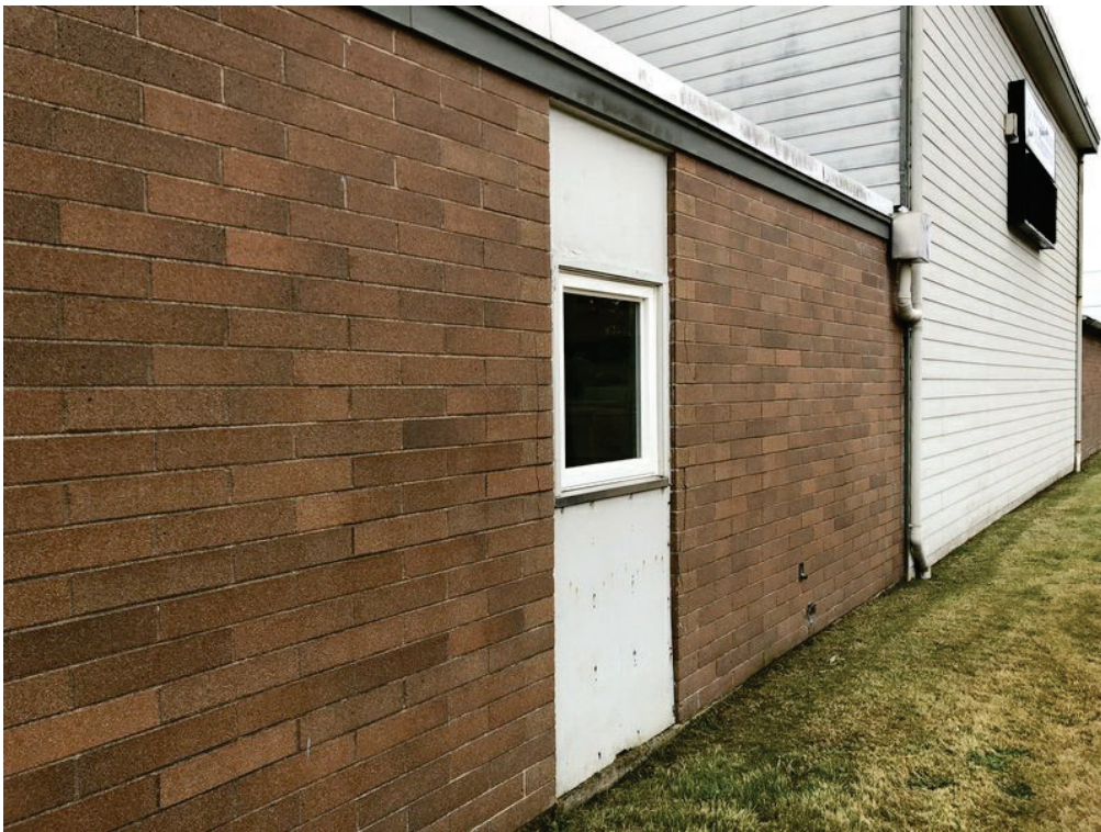
Figure 1-8. Brick walls at the North Elevation
