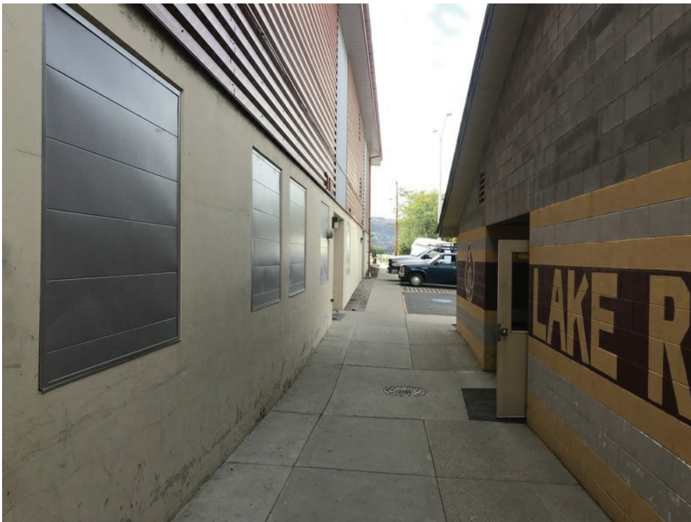
Figure 1-6. Separation between gymnasium building (on the left) and the wood shop (on the right).
