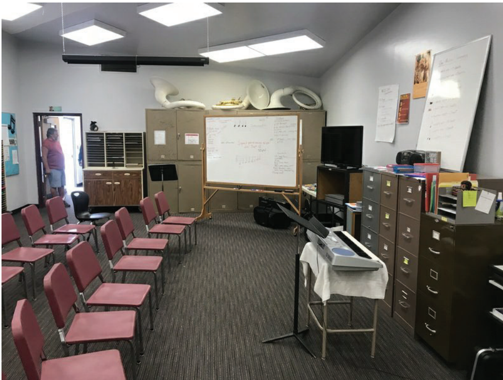
Figure 1-4. Band room with unsecured storage units and heavy instruments stored on top of units.
