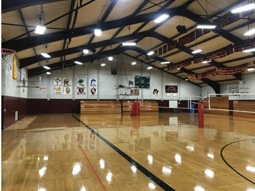
Figure 1-1. Interior view of gymnasium looking south.
