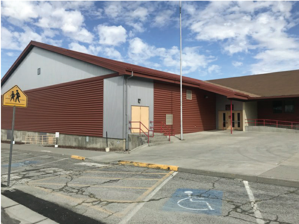
Figure 1-10. Exterior view from the southeast corner of the gymnasium, facing northwest.
