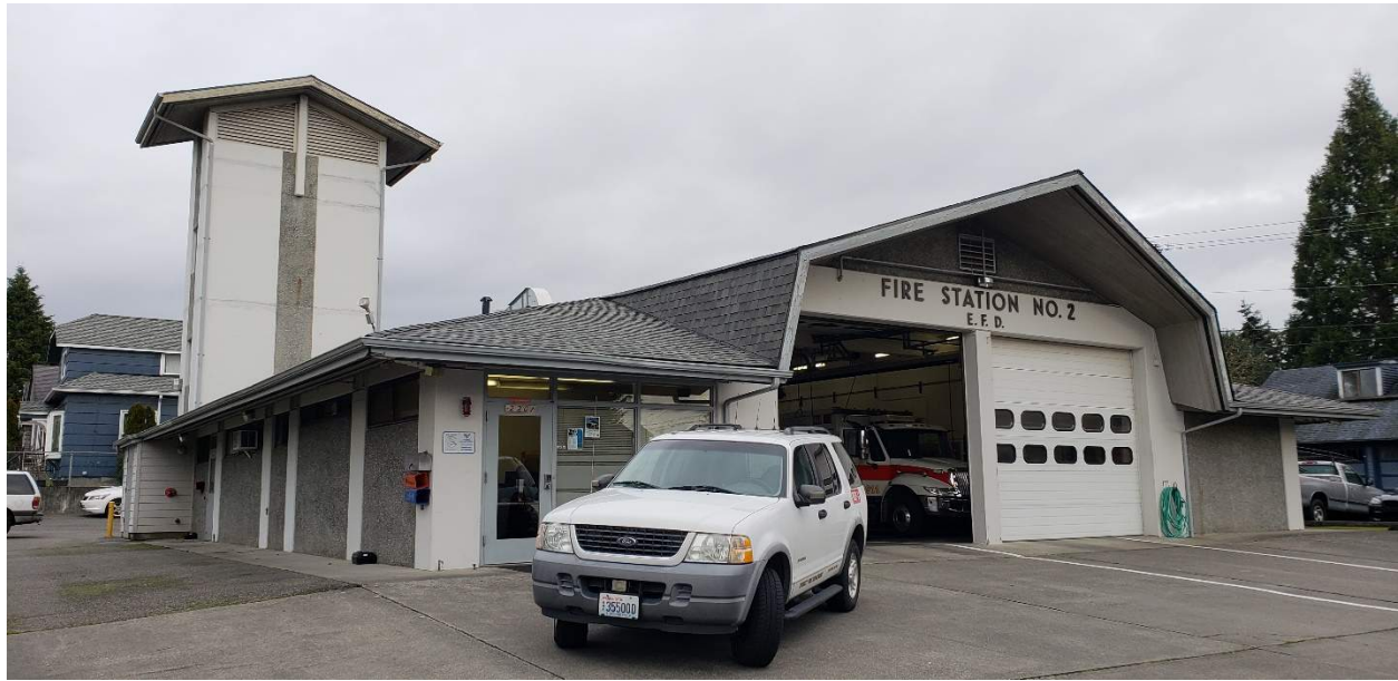
Figure 1-1. Everett Fire Station 2, Northwest Façade
