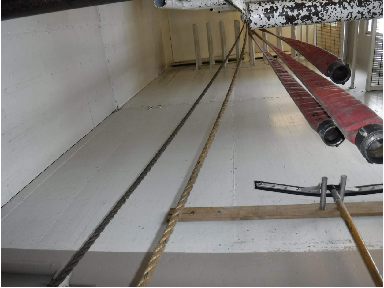
Figure 1-3. Everett Fire Station 2, Inside Hose Tower (Looking Up)
