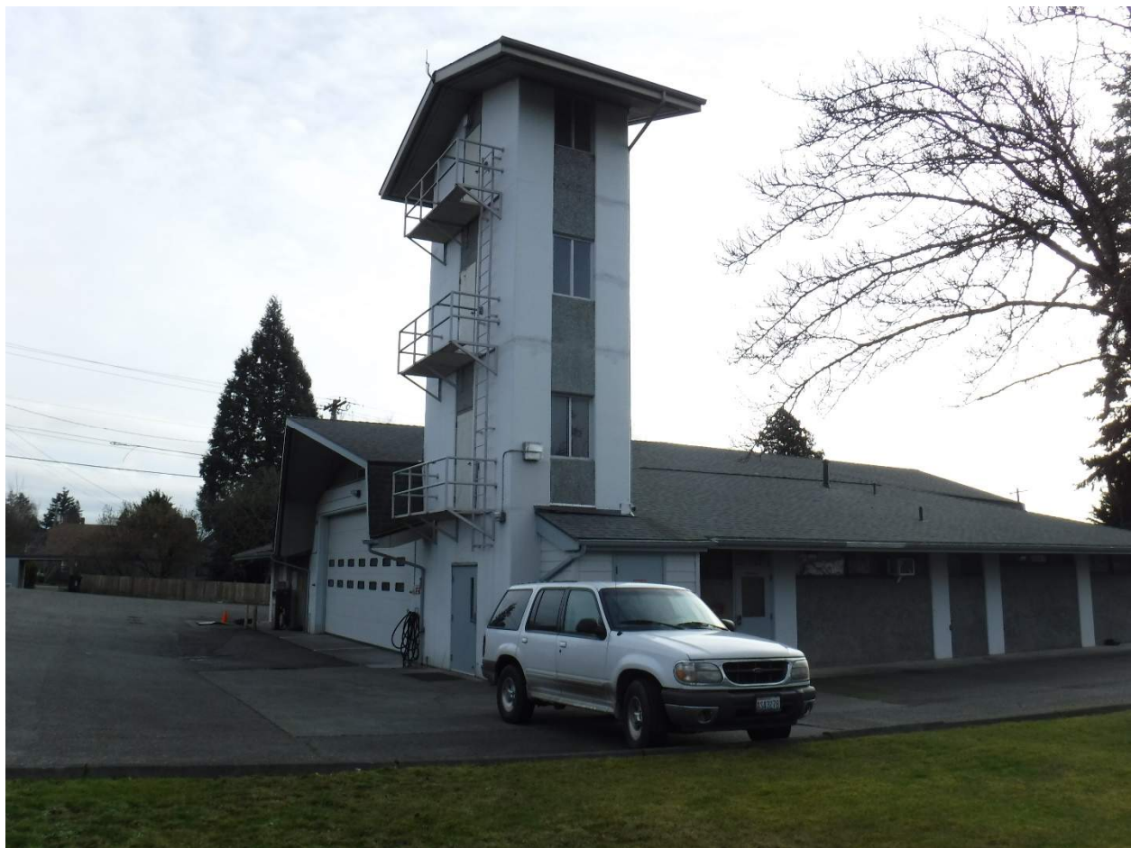
Figure 1-2. Everett Fire Station 2, Partial Northeast Façade
