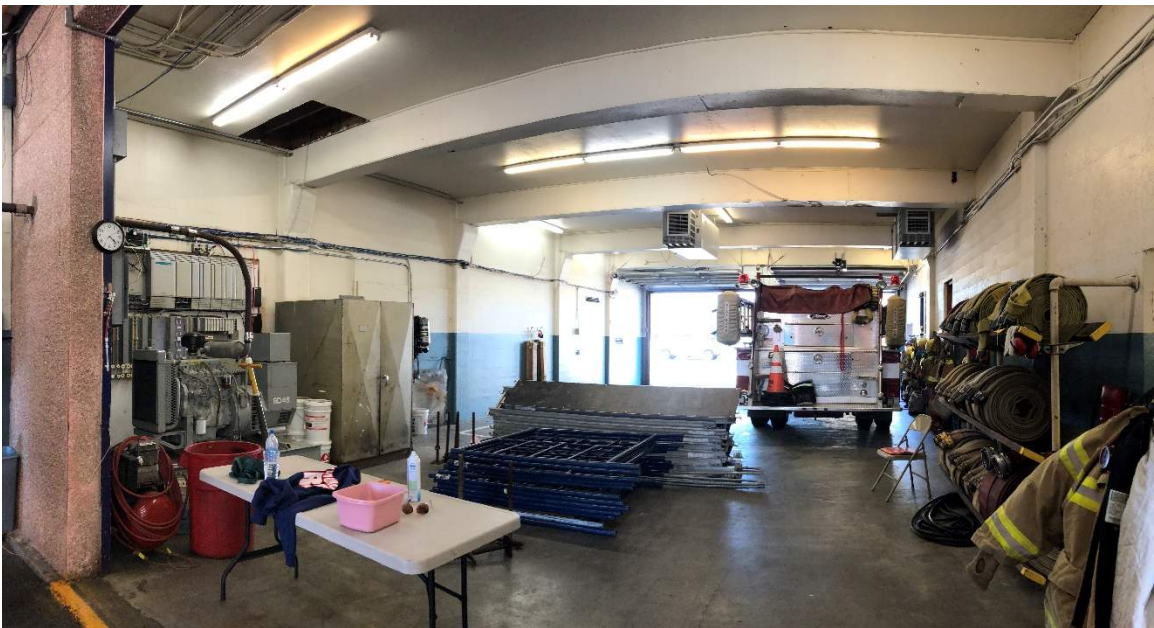
Figure 1-4. Typical Garage Bay
