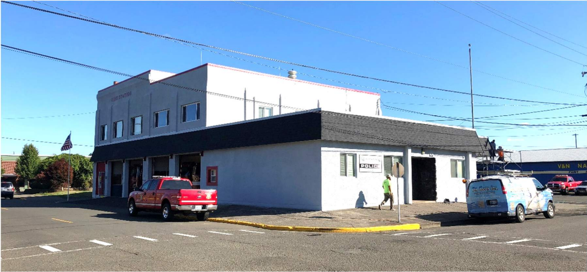
Figure 1-1. North West Exterior
