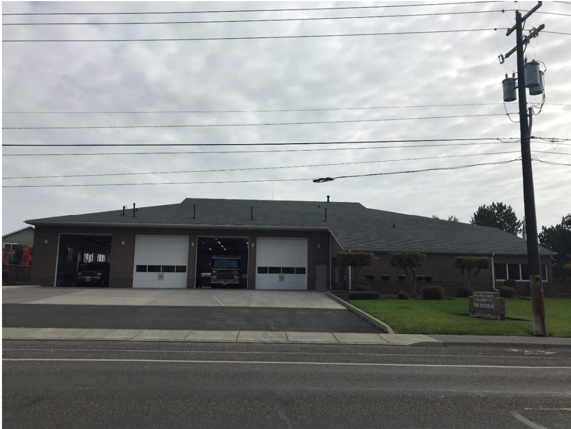
Figure 1-1. Walla Walla Station 41, West Facade
