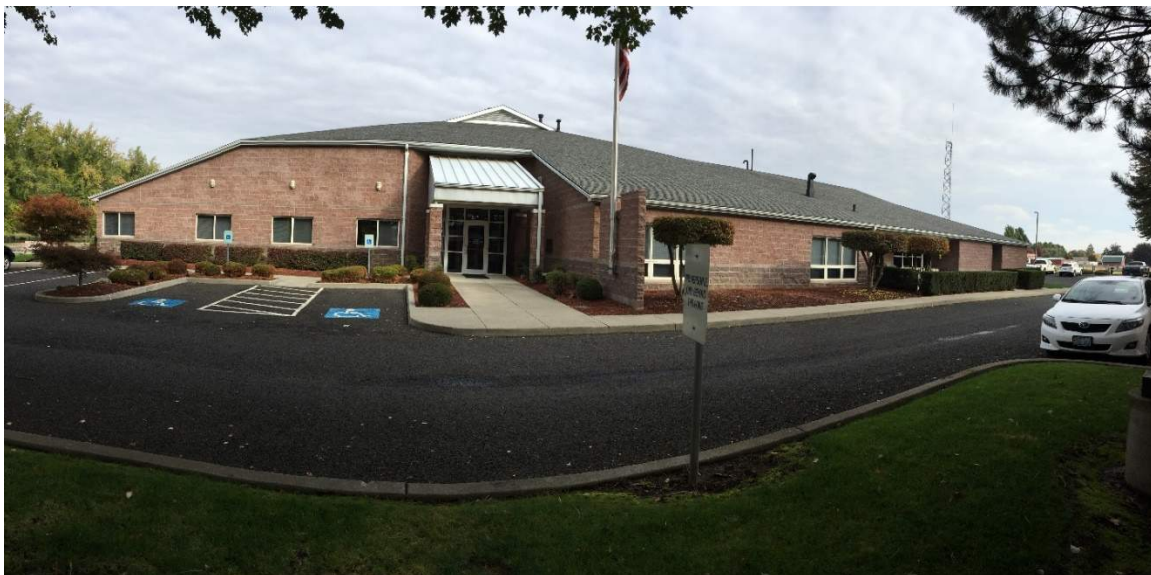
Figure 1-2. Walla Walla Station 41, South Facade
