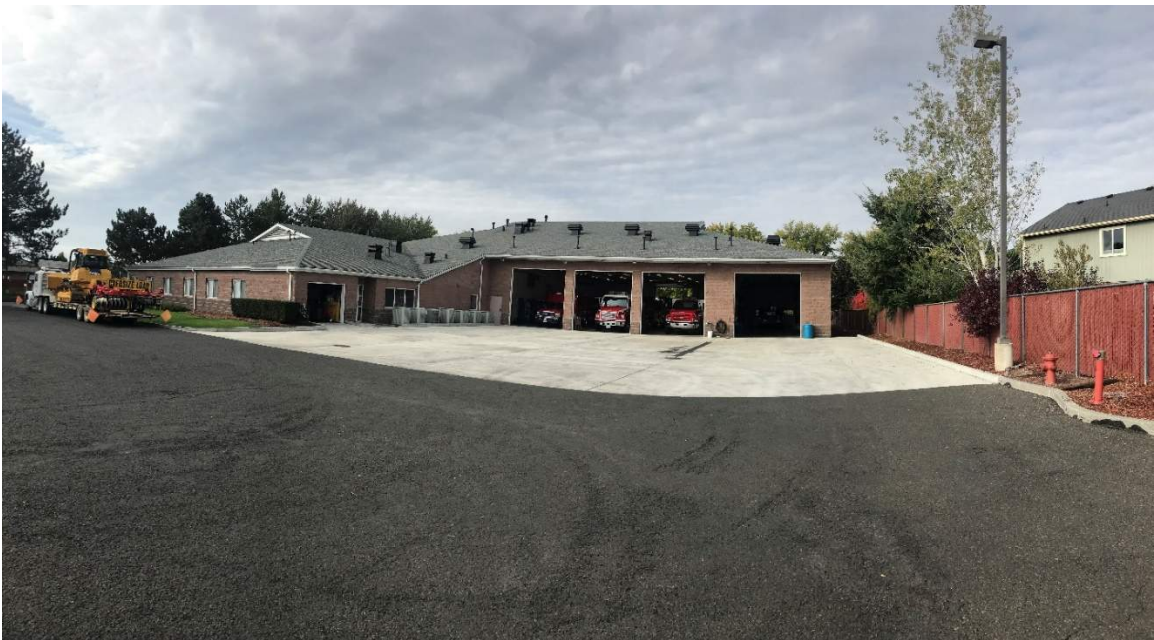
Figure 1-4. Walla Walla Station 41, South Facade
