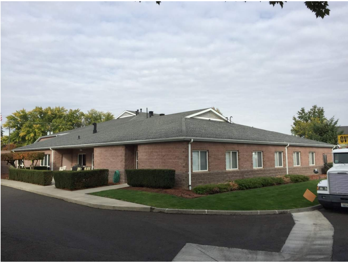
Figure 1-3. Walla Walla Station 41, Partial Southeast Facade
