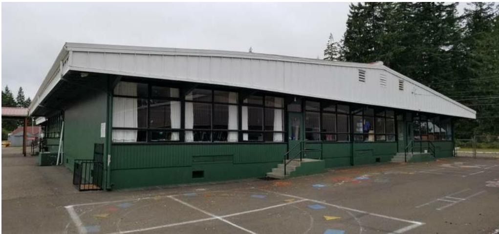
Figure 1-8. North façade of building.
