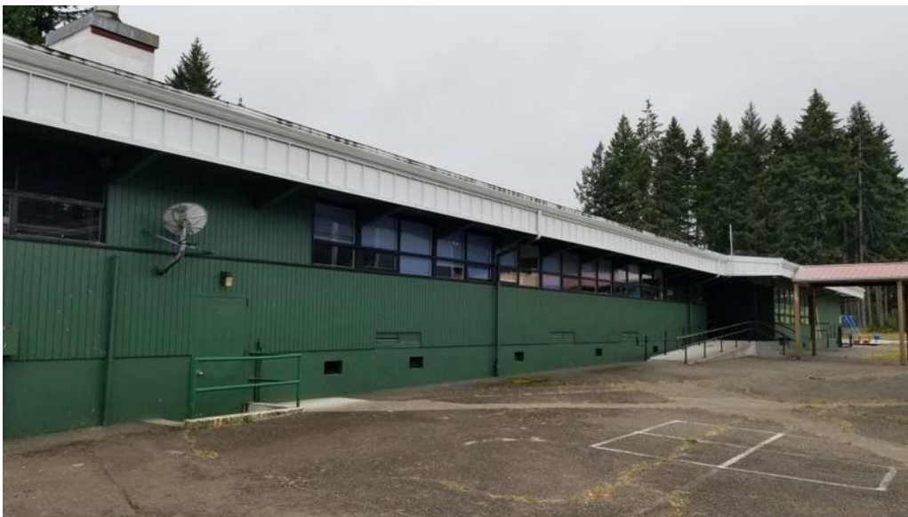
Figure 1-9. East façade of building.
