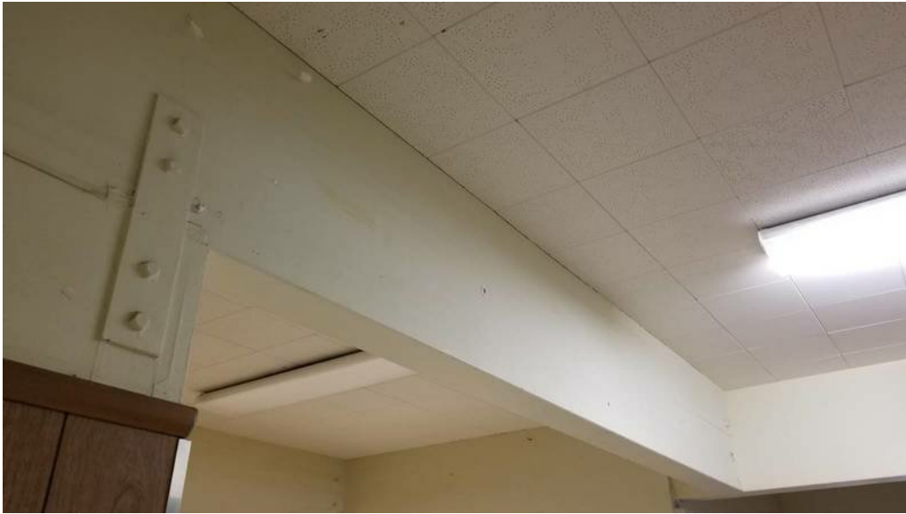
Figure 1-10. Exposed roof framing at interior.
