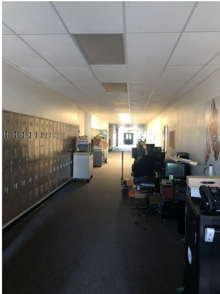
Figure 1-4. Suspended Ceiling in the Hallway
