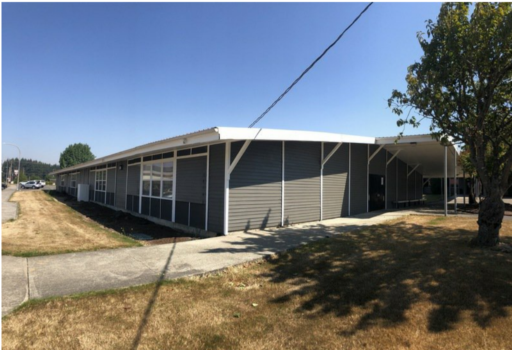
Figure 1-6. Building South Wall
