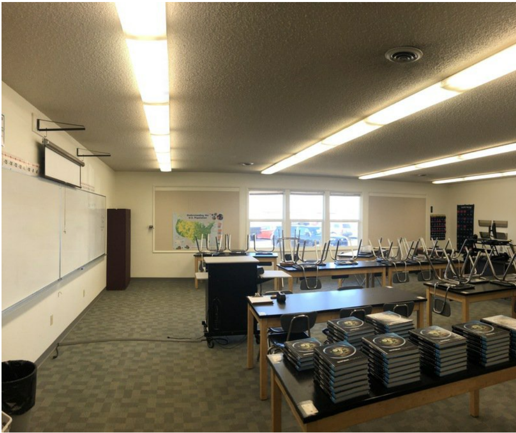
Figure 1-5. Gypsum Board Ceiling in a Typical Classroom
