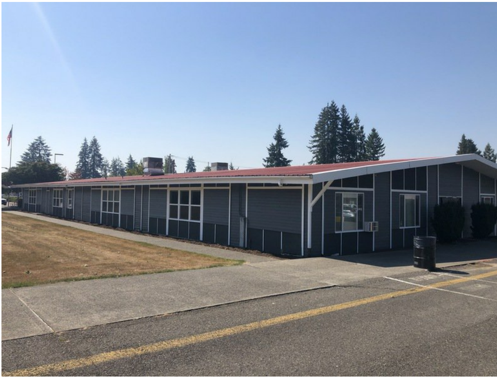
Figure 1-7. Building Exterior Wall
