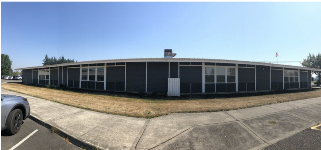
Figure 1-8. Building West Wall
