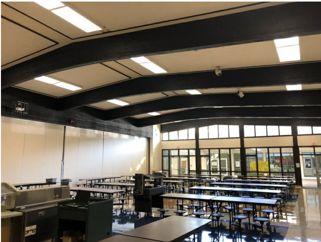
Figure 1-6. Cafeteria Showing Glulam Beam Roof Framing
