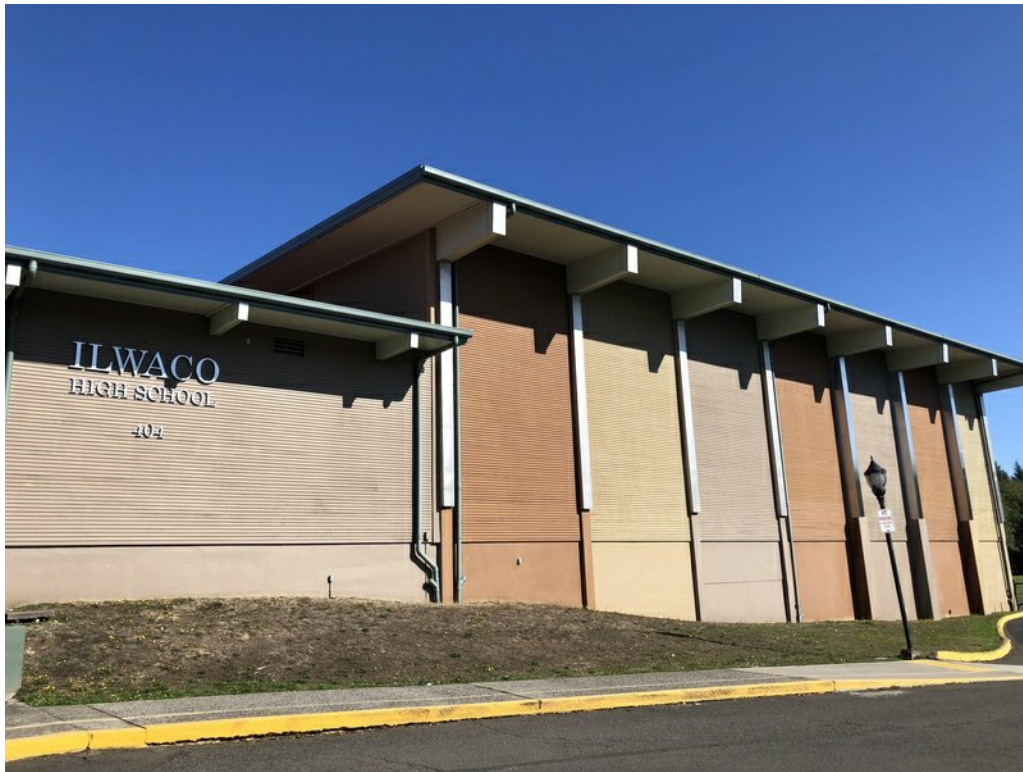
Figure 1-1. Ilwaco High School - South Exterior
