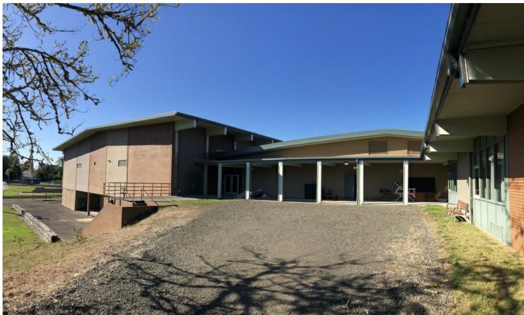
Figure 1-2. Ilwaco High School - East Exterior
