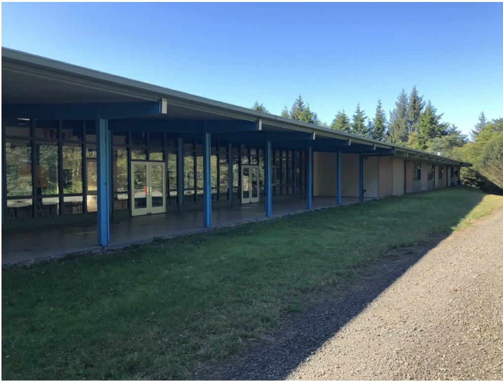
Figure 1-3. Ilwaco High School - North Exterior
