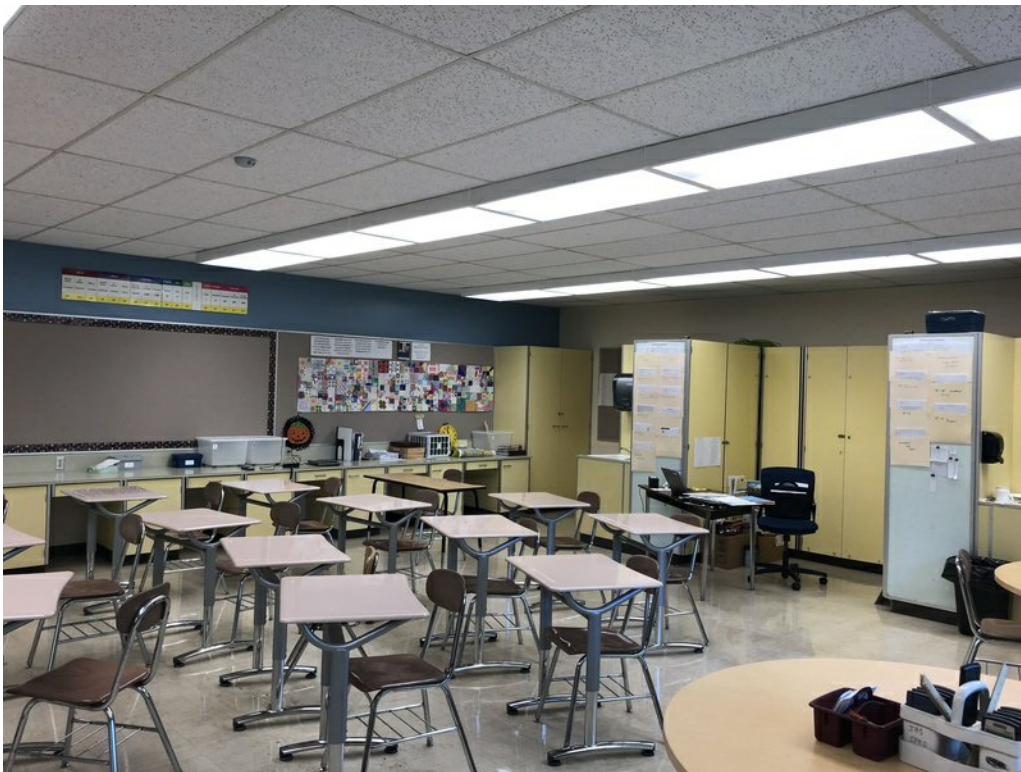
Figure 1-4. Typical Classroom with Tall Unbraced Cabinets
