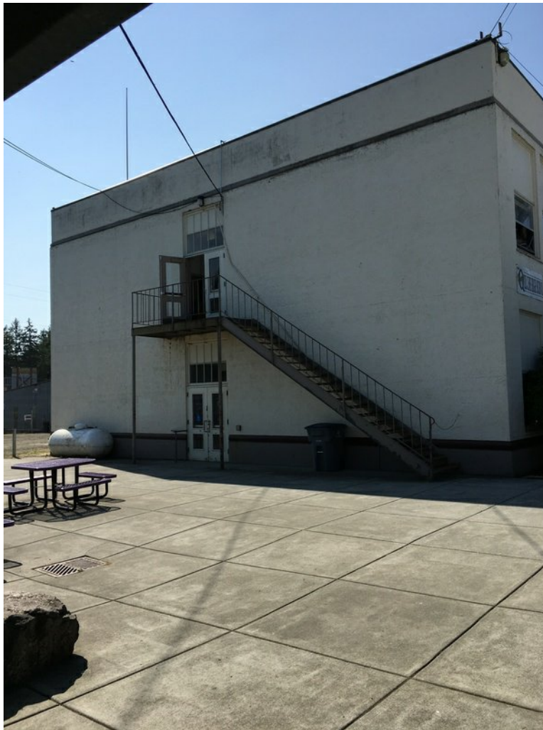
Figure 1-2. High School, North Elevation with Decommissioned Steel Stair
