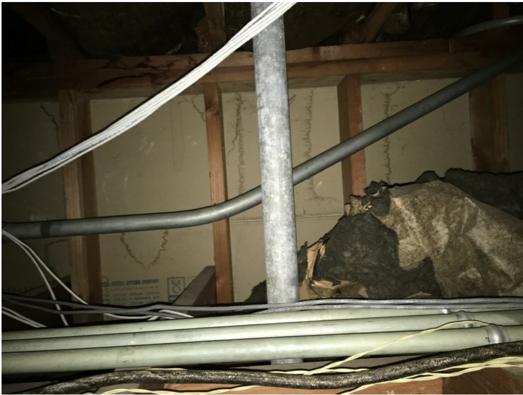
Figure 1-8. High School, Typical Framing Above Ceiling
