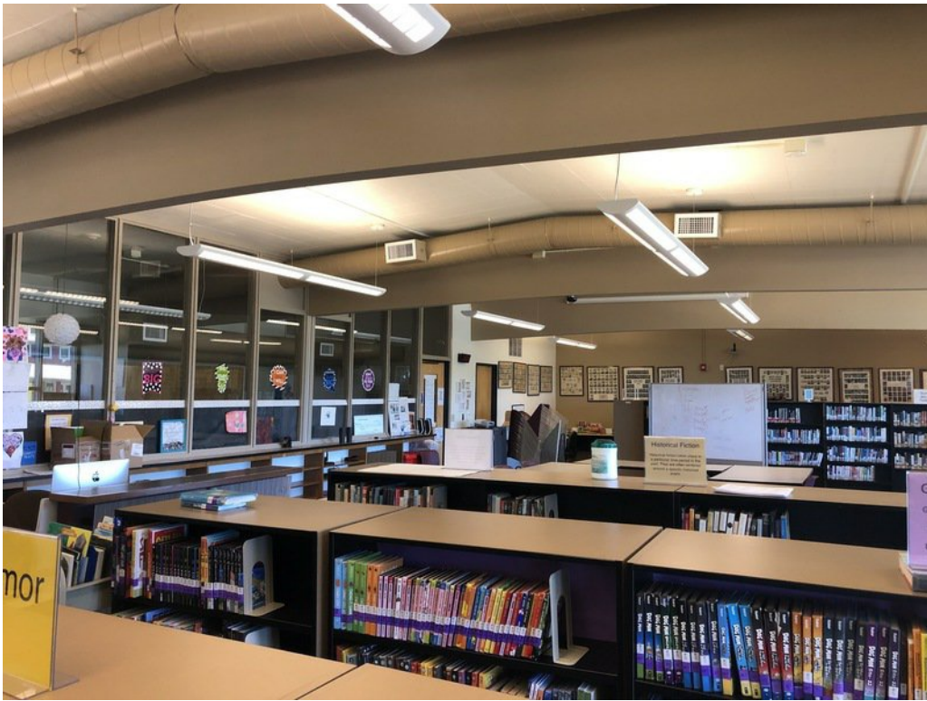
Figure 1-7. Roof Framing in Library
