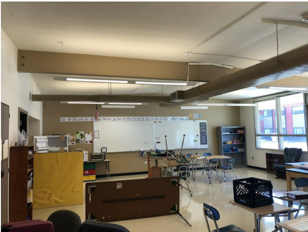
Figure 1-6. Roof Framing in Classroom
