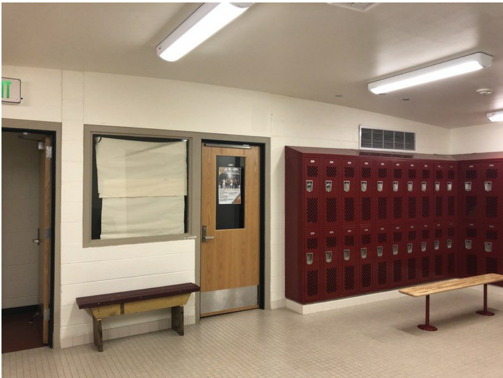
Figure 1-8. CMU Walls in Locker Room
