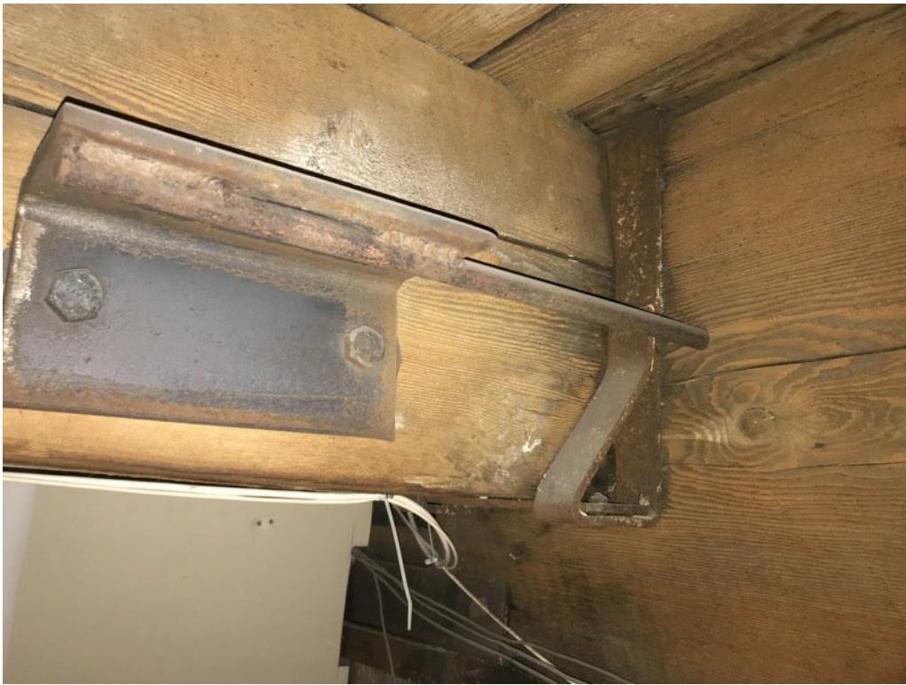
Figure 1-7. Joist to girder connection at the interior mechanical space.
