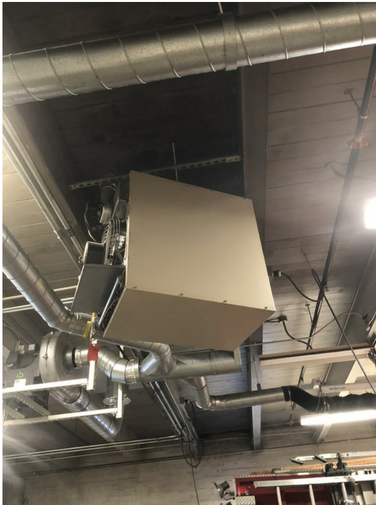
Figure 1-4. Figure-4 Apparatus Bay Roof Framing, Mech. Unit & Ducts
