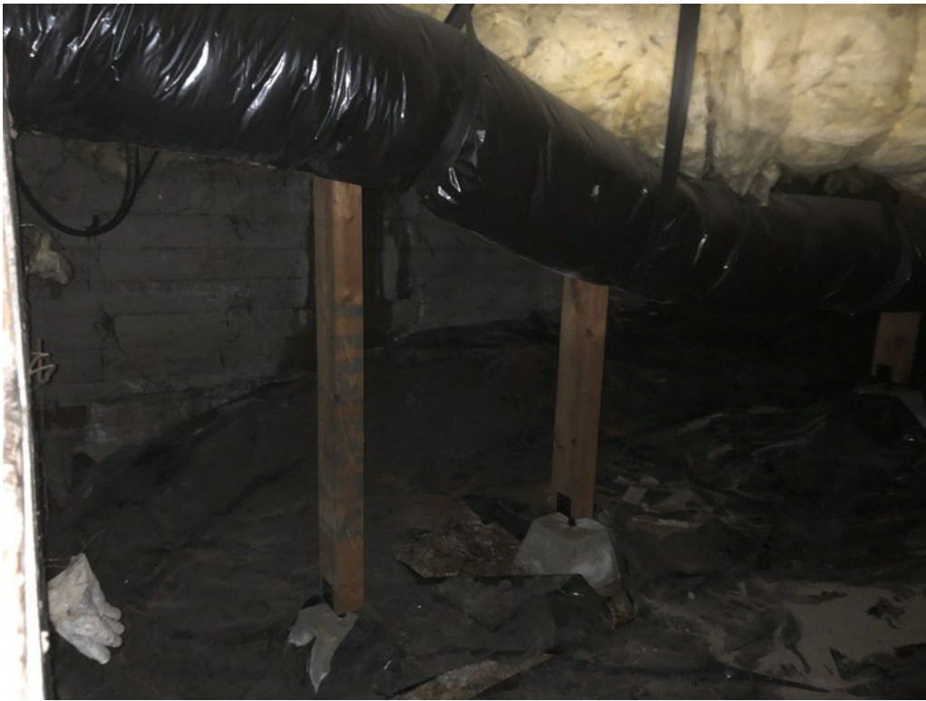
Figure 1-7. Figure-7 Floor Framing at Crawl Space Under Living Quarters
