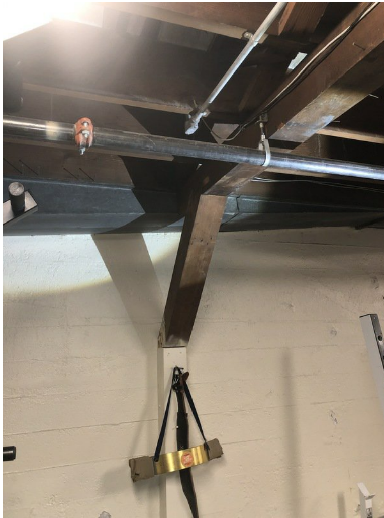
Figure 1-6. Figure-6 Basement Floor Framing & Ducts at Periphery to Concrete Wall
