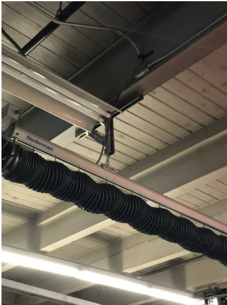
Figure 1-5. Figure-5 Apparatus Bay Roof Framing & Tracks at Hose Pipe
