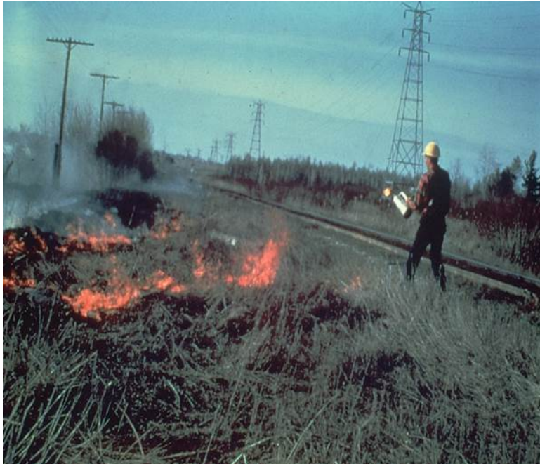
Figure 123. Right-of-way maintenance burning.
