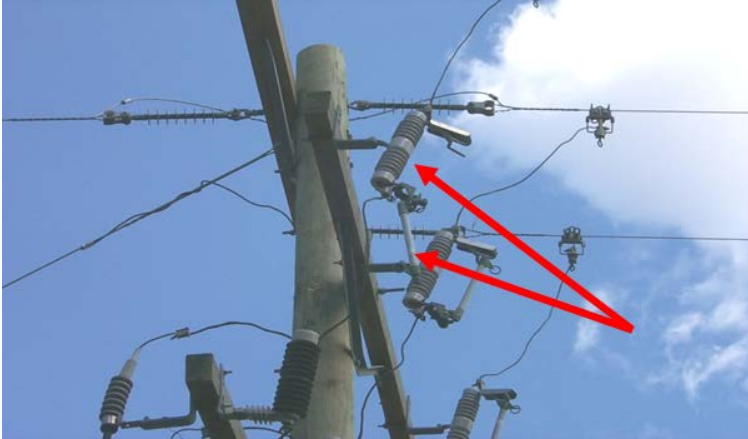
Figure 139. Solid blade disconnect.
