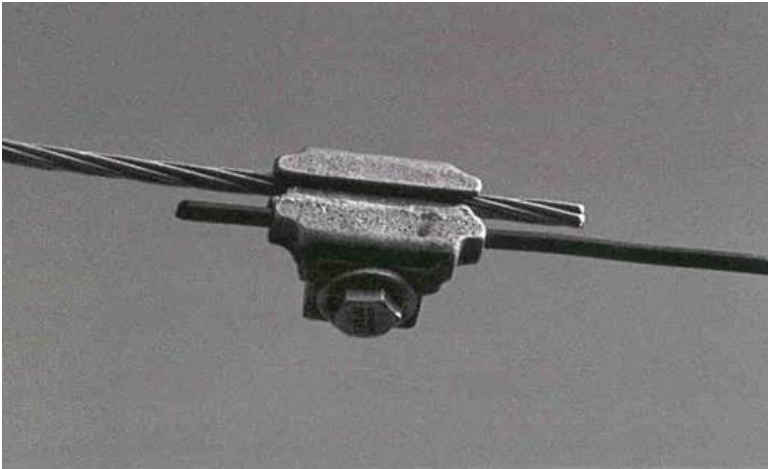
Figure 147. LM connector.
