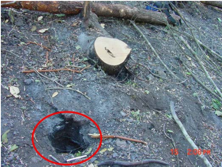
Figure 135. Blowhole near tree from electrical grounding.
