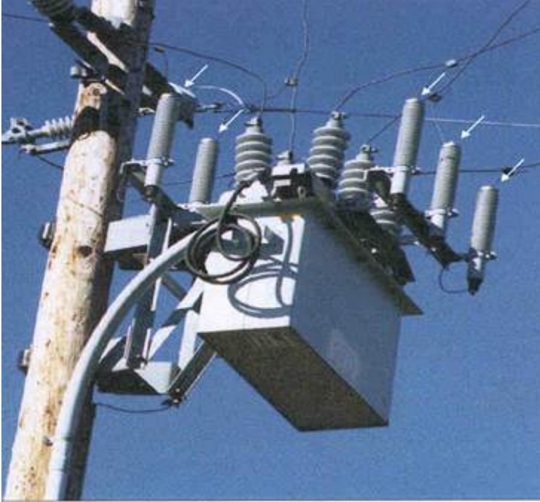
Figure 141. Lightning arresters.
