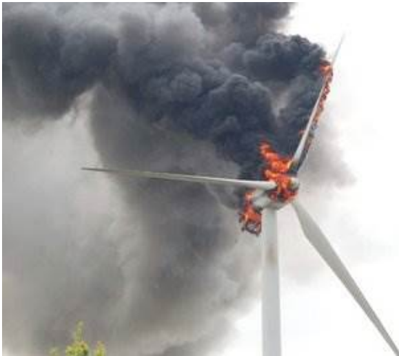
Figure 183. Wind turbine fire.
