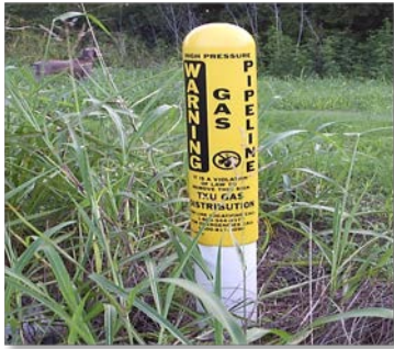
Figure 78: Natural gas pipeline road crossing marker
