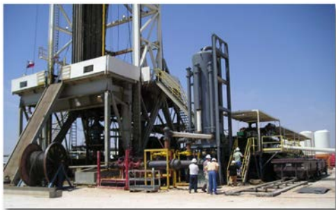
Figure 94: Drilling rig floor with vertically stacked drill pipe
