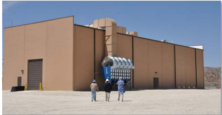
Figure 30: Building housing Presidio battery
