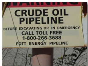
Figure 57: Crude oil pipeline road crossing marker
