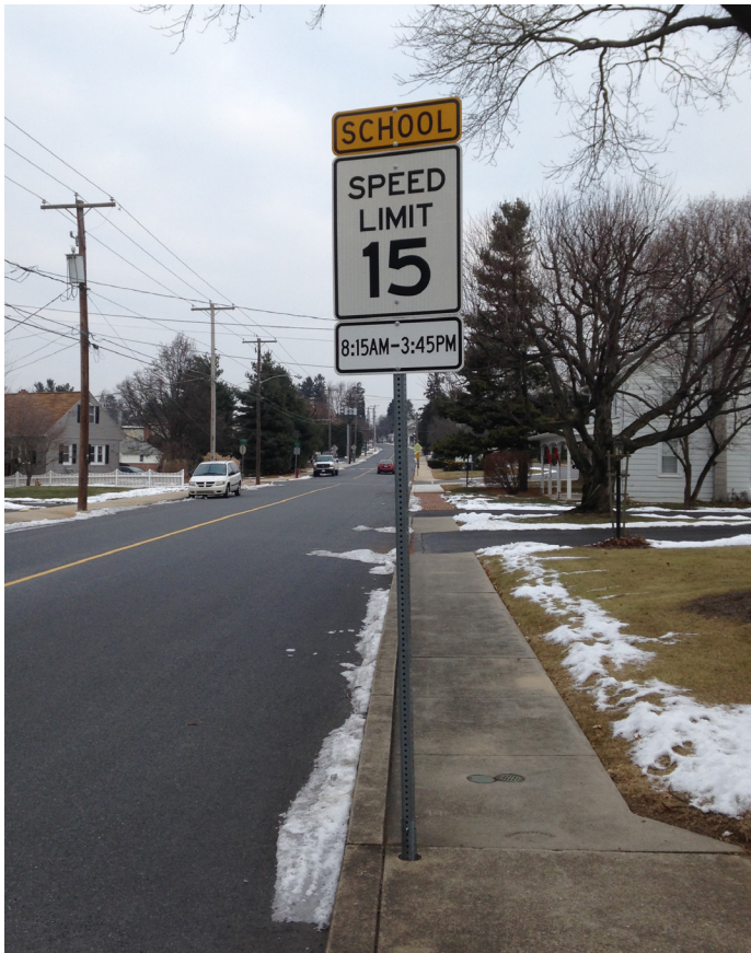
Speed limits can be lowered for a school zone for the times of the day when students would be traveling to and from school. This is a school speed limit sign assembly. Photo: PennDOT LTAP
