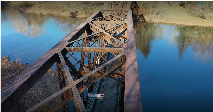
A drone image from above a truss bridge. Photo: NTM Engineering
