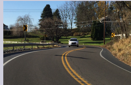
Centerline rumble strips are a proven safety countermeasure intended to alert drivers when they leave the roadway through the generation of noise and vibration. Photo: PennDOT STIC
