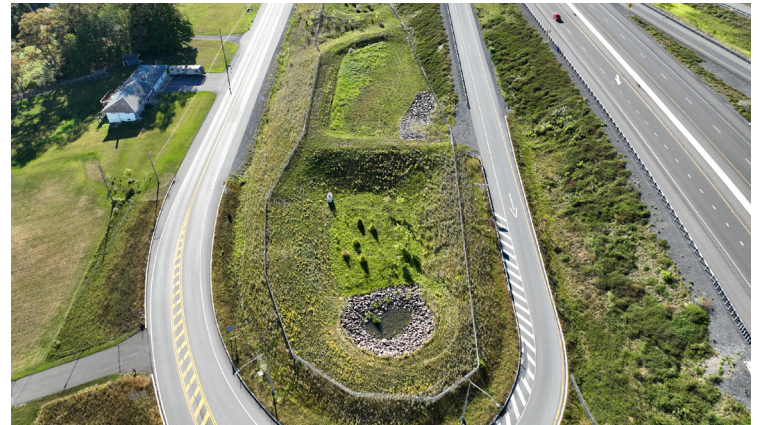
Drone imagery for a stormwater basin inspection. Photo: NTM Engineering
