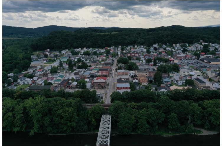
A drone photograph of Newport Borough in Perry County. Photo: NTM Engineering
