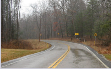
Installation of curve warning signs on rural roads alerts drivers and helps them navigate the roadway safely. Photo: PennDOT STIC
