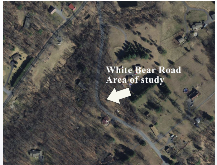
Figure 1: An aerial view of the study area. Photo: PennDOT/PEMA
