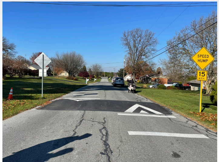
Stanton Road after the new signs were installed. Photo: PennDOT LTAP
