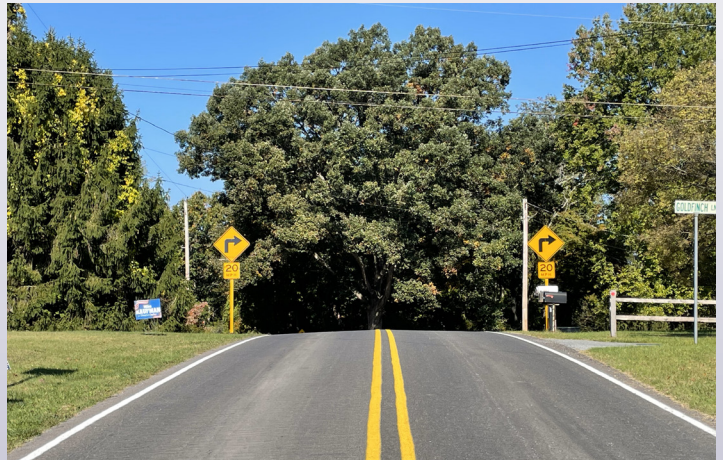
Figure 3: New warning signs were among the improvements implemented by the township. Photo: PennDOT LTAP
