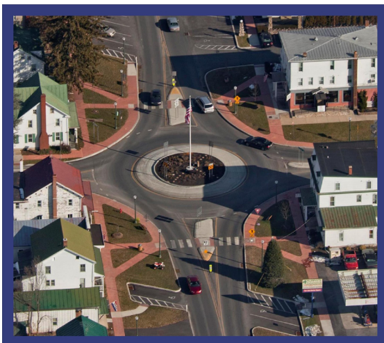
Linglestown Roundabout / Linglestown Road (PA-39)
