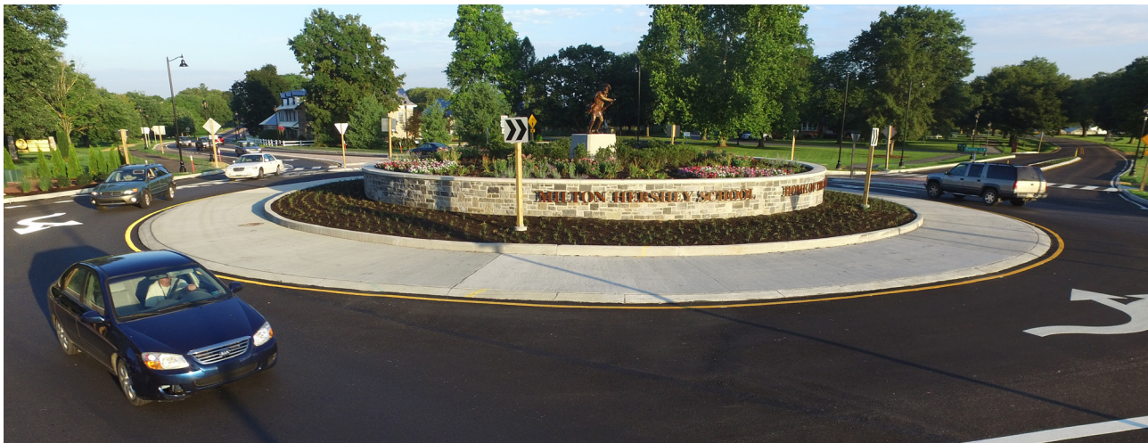
An example of aesthetic roundabout treatments can be seen in this image taken near Milton Hershey School. Photo: Pennoni and Milton Hershey School
