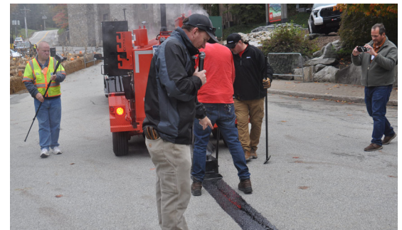
Mastic was demonstrated to repair a larger crack. Photo: Mid-Atlantic RMC
