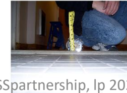
100_2205 Hyattsville Municipal Building
