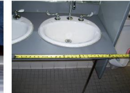
100_2207 Hyattsville Municipal Building
