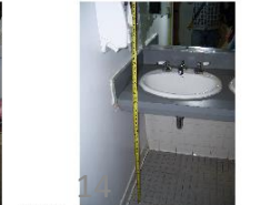
100_2208 Hyattsville Municipal Building
