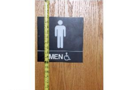
100_2204 Hyattsville Municipal Building
