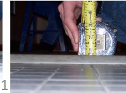
100_2206 Hyattsville Municipal Building
