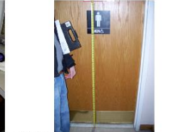
100_2203 Hyattsville Municipal Building
