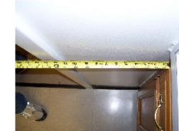
100_2201 Hyattsville Municipal Building
