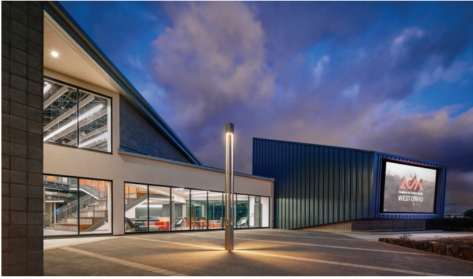
Outside the new Academy for Creative Media West O'ahu building. The high tech 33,000-square-foot facility features the latest video, graphics, animation, social media, web and app development equipment and rooms.
