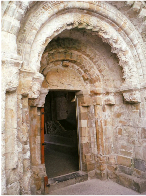
North doorway to chapel
