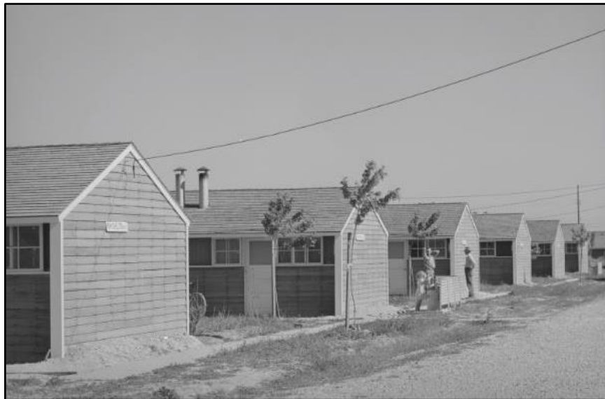
Figure 3-19. The barracks-style buildings at the Caldwell camp, 1941. Library of Congress, Prints & Photographs Division, FSA-OWI Collection, LC-USF34-039194-D.
