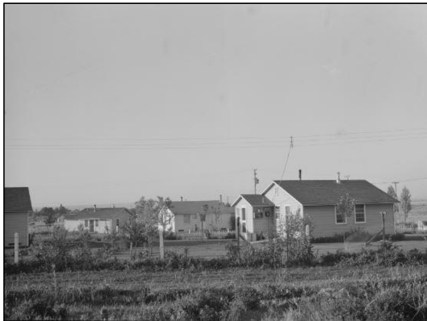
Figure 3-5. The camp had forty-seven small houses or cottages. Each house had a kitchen, living/dining room, two bedrooms, and a bathroom. Library of Congress, Prints & Photographs Division, FSA-OWI Collection, LC-USF34-073761-D.
