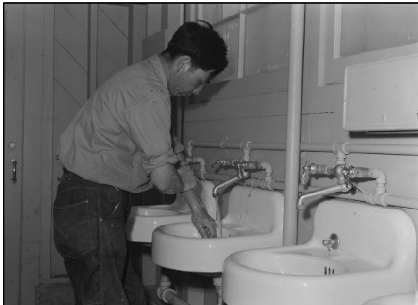
Figure 3-8. The apartments in the barracks-style building lacked indoor plumbing. Camp residents used comfort stations located between the rows of barracks. Library of Congress, Prints & Photographs Division, FSA-OWI Collection, LC-USF34-073758-D.
