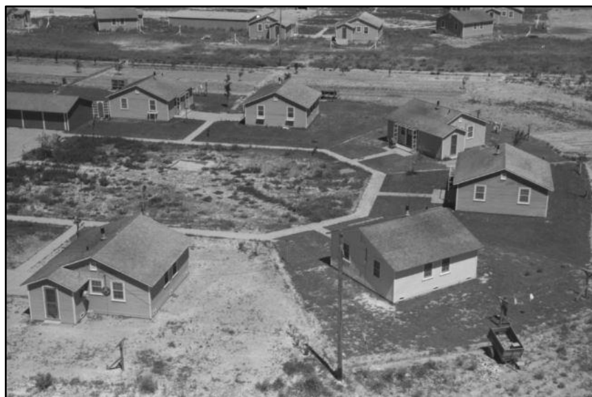
Figure 3-17. The small houses at the Caldwell camp, photographed in 1941, were similar in style to those at the Twin Falls camp. Library of Congress, Prints & Photographs Division, FSA-OWI Collection, LC-USF33-013032-M4.
