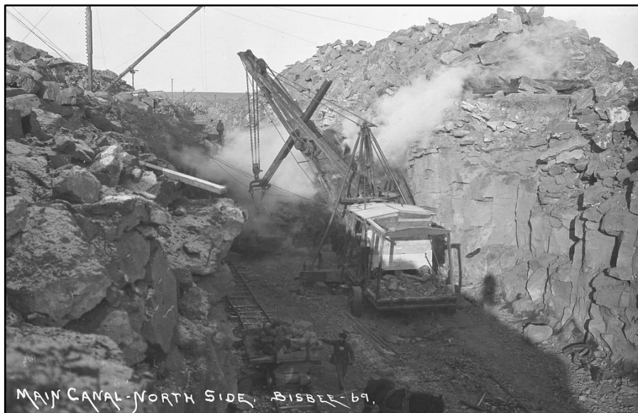
Figure 1-1. A steam shovel digs the North Side Canal from Milner Dam, ca. 1906. Twin Falls Public Library, Clarence E. Bisbee Collection, PC-2084.
