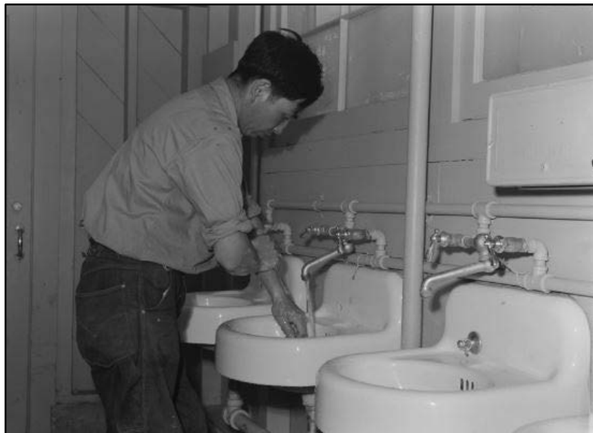
Figure 3-8. The apartments in the barracks-style building lacked indoor plumbing. Camp residents used comfort stations located between the rows of barracks. Library of Congress, Prints & Photographs Division, FSA-OWI Collection, LC-USF34-073758-D.
