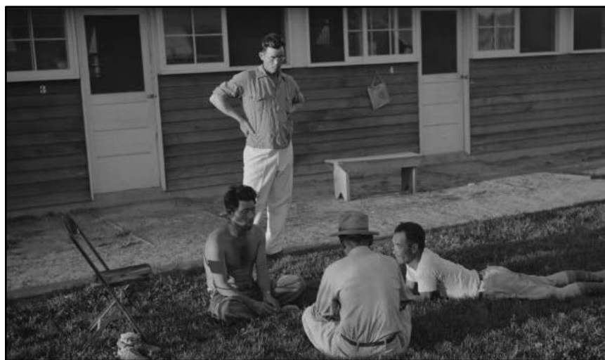
Figure 3-12. Beginning in 1942, the Twin Falls labor camp was occupied primarily by single Japanese American men. As the War Relocation Authority began to encourage family unit resettlement away from the concentration camps, an increasing number of Japanese American families began to reside in the camp. Library of Congress, Prints & Photographs Division, FSA-OWI Collection, LC-USF34-027753 D
