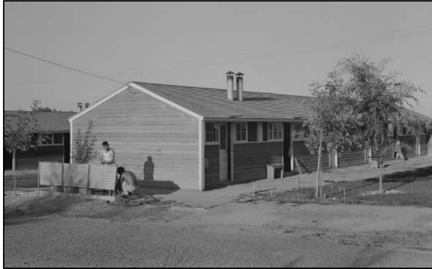
Figure 3-20. The barracks-style buildings at the Twin Falls camp, pictured in 1942, are nearly identical to those at the Caldwell camp. Library of Congress, Prints & Photographs Division, FSA-OWI Collection, LC-USF34-073767-D.
