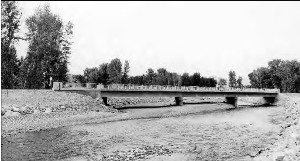
Figure 79. The Big Wood River Bridge, pictured in 1957, was the first use of prestressed-concrete girders in Idaho.
