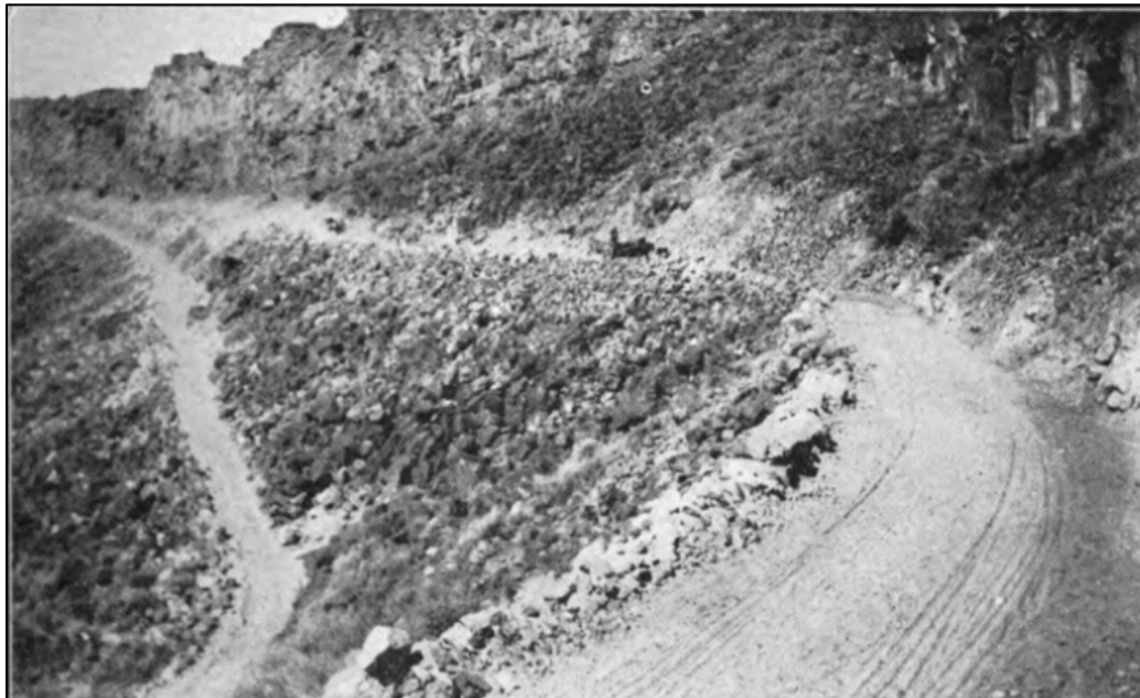
Figure 27. Comparison between old road (at left) and new standard construction of the Sawtooth Park Highway, Lincoln County, 1914. 188
