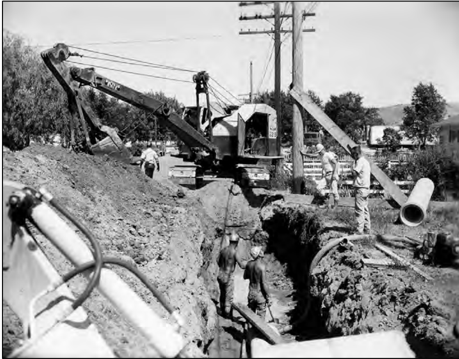
Figure 110. Road construction in Payette in 1966. 553
