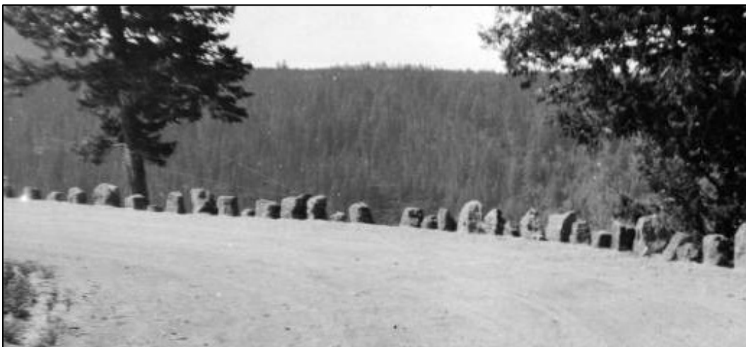
Figure 41. Lava rock guardrail on Warm River-Yellowstone Road (ID-47). 267
