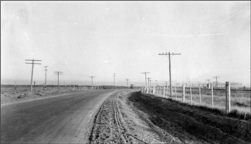
Figure 32. Typical highway construction on the Yellowstone Park Highway in Bingham County in 1923 showing an early type of bituminous surface treatment, 18-foot roadway, gravel shoulders, and ditches. 198
