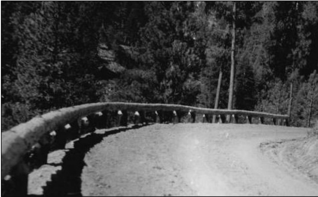
Figure 42. Log guardrail built in 1924 on North Fork-Payette Highway, Boise County. 268
