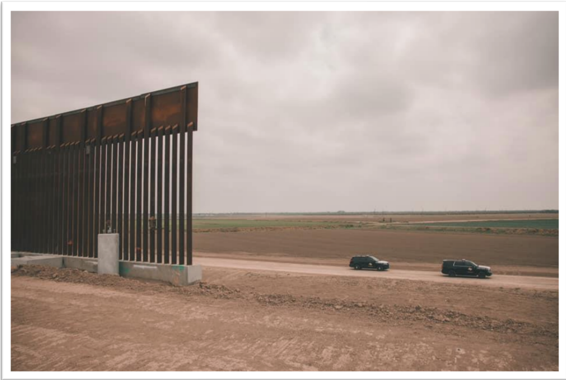
A section of unfinished border wall in the Rio Grande Valley Sector, Texas, in March 2021. (Source: HSGAC subcommittee report on canceled border wall construction)
