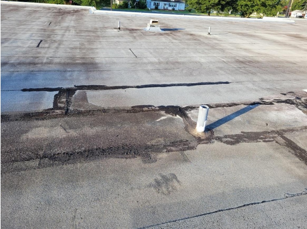
Typical roof repair in failing roof system.
