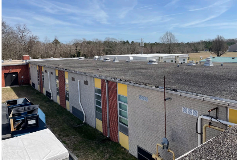
EXISTING ROOF / WINDOWS
