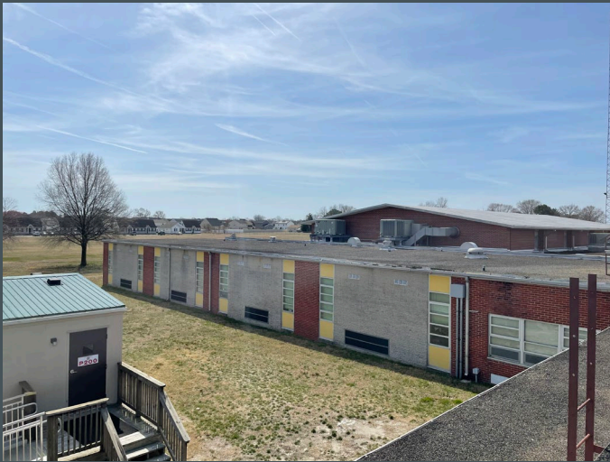
EXISTING BUILDING ENVELOPE
