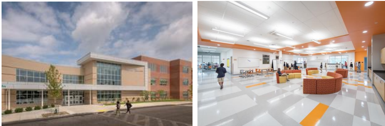
Photos courtesy of Grimm + Parker Architects; Photo credit: Sam Kittner; Fort Worthington exterior and collaborative area
