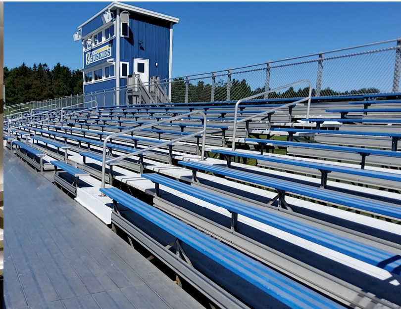
Northern High, Garrett County
