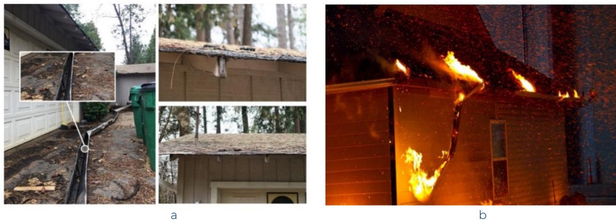
Figure 1. Direct flame contact to the edge of the roof caused by ignited debris in the gutters during ember storms (a) in the Camp Fire (2018) in County, California (home defended by first responders), and (b) a vinyl gutter melts off a house during testing at the IBHS Research Center.
