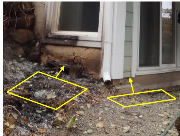
Figure 5a-b. Example of vegetation in small amounts located in Zone 0 creating a pathway for fire spread: (a) Wood mulch provided a pathway for fire to get close to the building and ignite a hot tub during the Glass Fire (2020) in Napa and Sonoma Counties, California; (b) Ground-level plants during the Glass Fire (2020).
