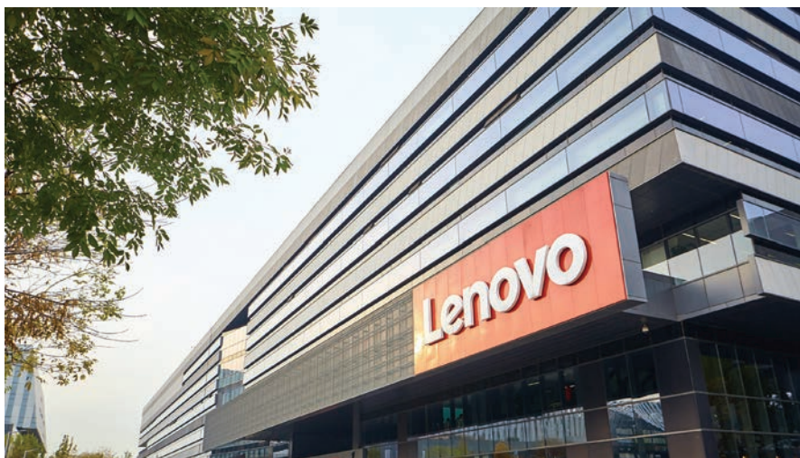
Lenovo's operation center in Beijing, China.
