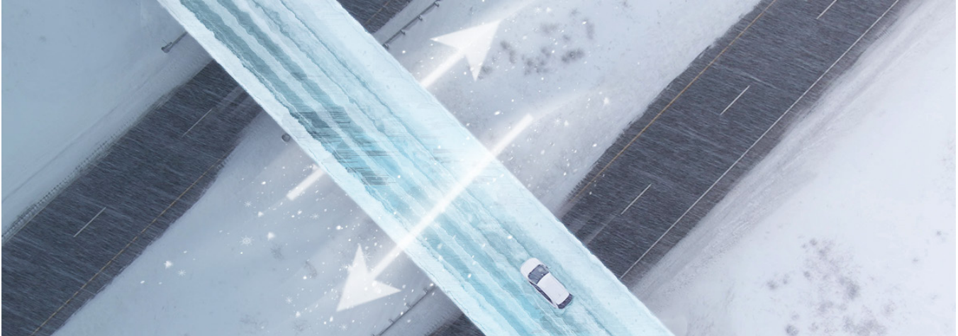
Figure 5.10: Ice forms on bridges first due to circulating air both above and below the road surface.
