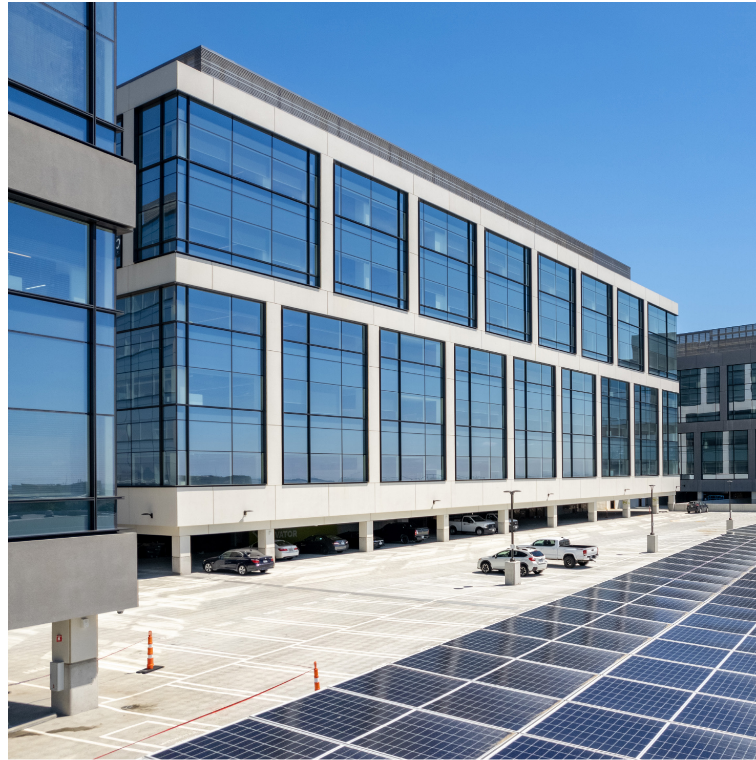
Solar Panels Installed on Garage at Kilroy Oyster Point – LEED Gold
