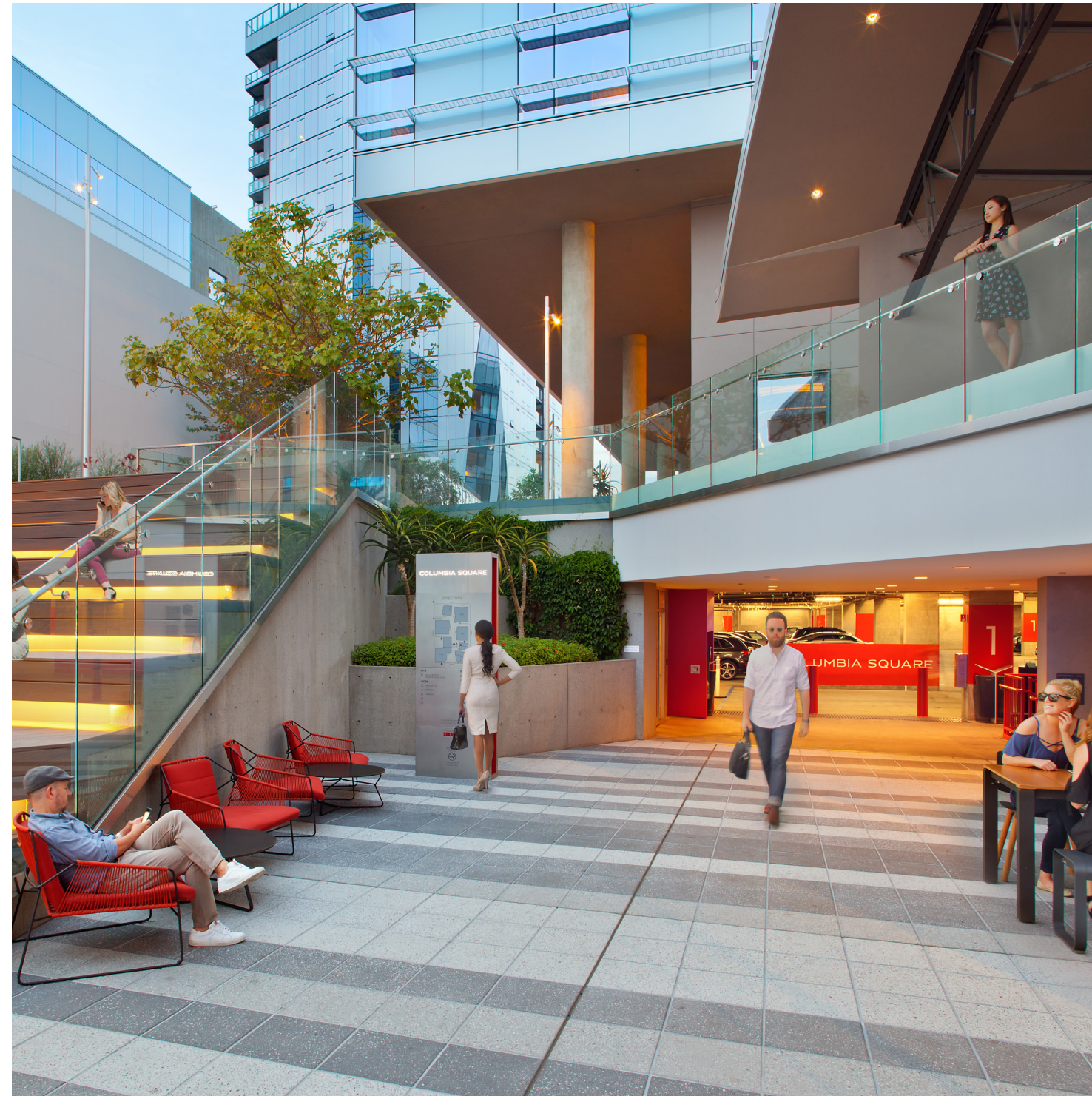
Columbia Square, Los Angeles, CA - LEED Gold, WELL Silver, WELL Health-Safety, Fitwel, ENERGY STAR
