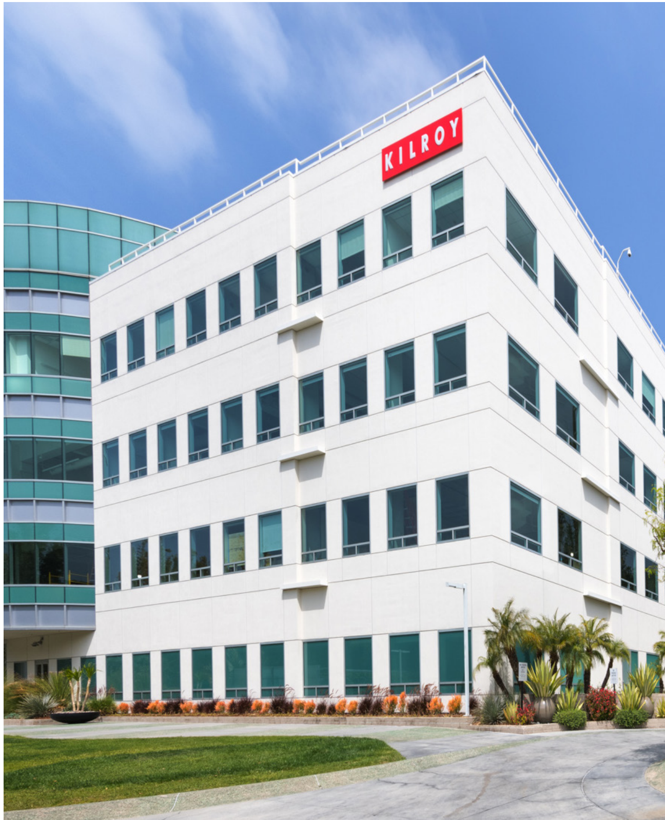
Westside Media Center, Los Angeles, CA – LEED Silver, Fitwel, WELL Health-Safety, ENERGY STAR
