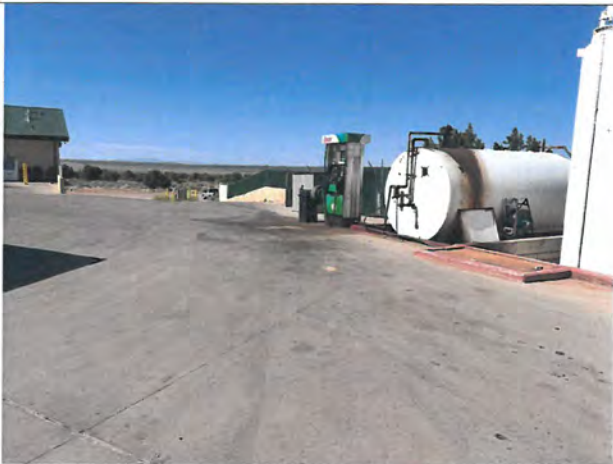
Photo 33 - Diesel fuel pump with stained and over-spilled fuel on concrete surface
