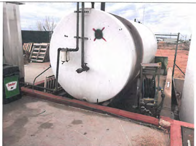
Photo 34 - Diesel fuel above ground storage tank on an adjacent property
