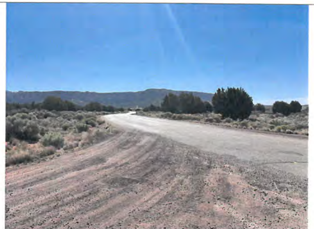
Photo 6 - Looking East along Arizona Ave. from corner of Arizona Ave. and Redwood St.
