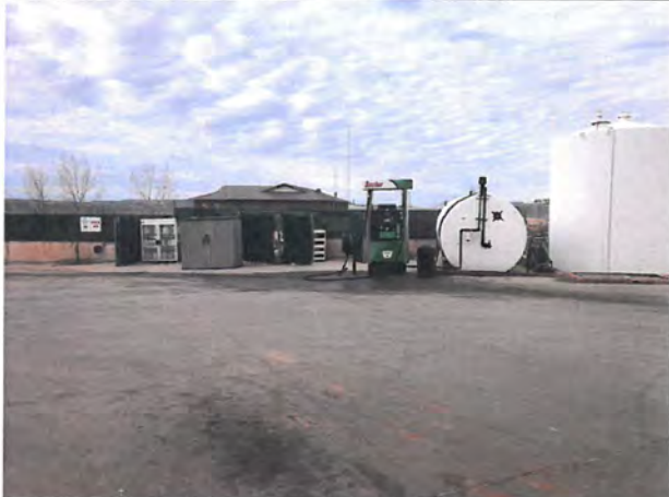
Photo 35 - Diesel fuel pump with stained and over-spilled fuel on concrete surface
