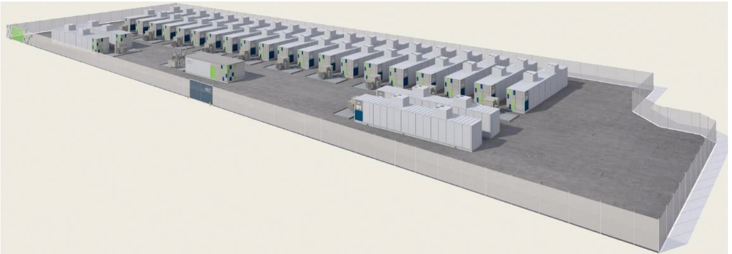
Figure 5: Typical 30 MW, 120 MWh Lithium-Ion Energy Storage Site 13
