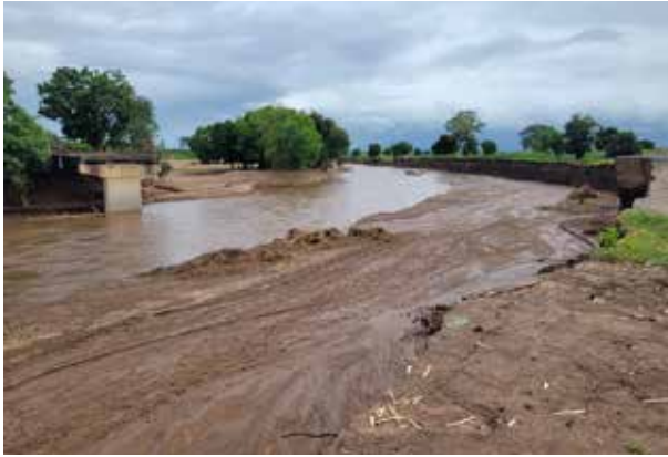
Collapse of bridge on M1 road, Chikwawa. (World Bank mission team; WFP Drone Imagery)
