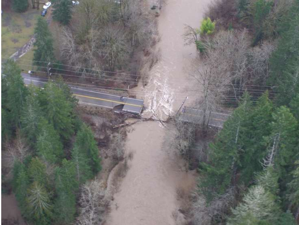
Figure 8-9 Belfair-Tahuya Bridge on the Tahuya River December 2007 (DR 1734)
