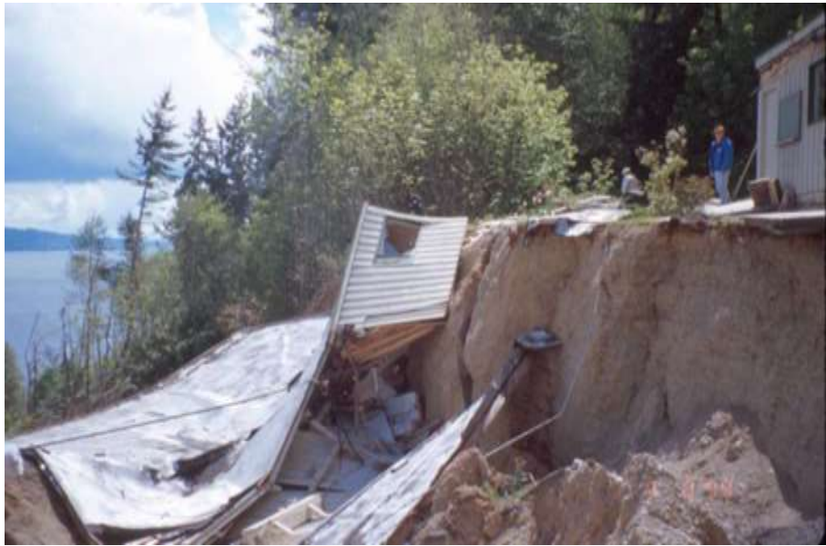
Figure 9-5 House destroyed by landslide in Lilliwaup during 1998-1999 winter
