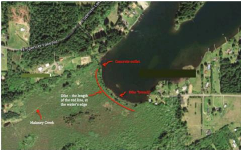
Figure 6. Dike and outlet at southwest end of Spencer Lake
